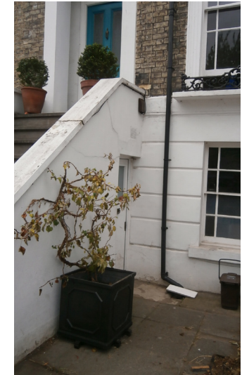
Door on side of external stairs
