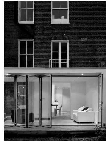
Maida Vale Wilkinson King Architects AJ Robin Ellis Small Project Award, 1998 Sympathetic extension with full height glazing
