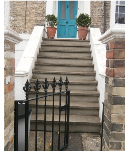
Front gate and steps to small porch and front door
