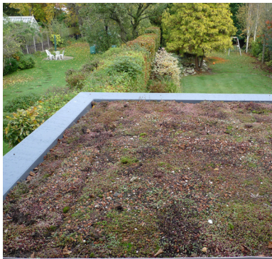
Harpenden Wilkinson King Architects Sedum roof
