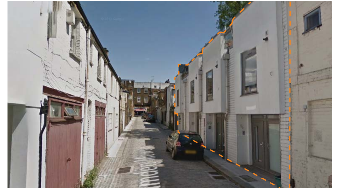
Figure 13. Street view showing 2.5 storey buildings at 96 - 102 Camden Mews. Highlighted on right of image.
