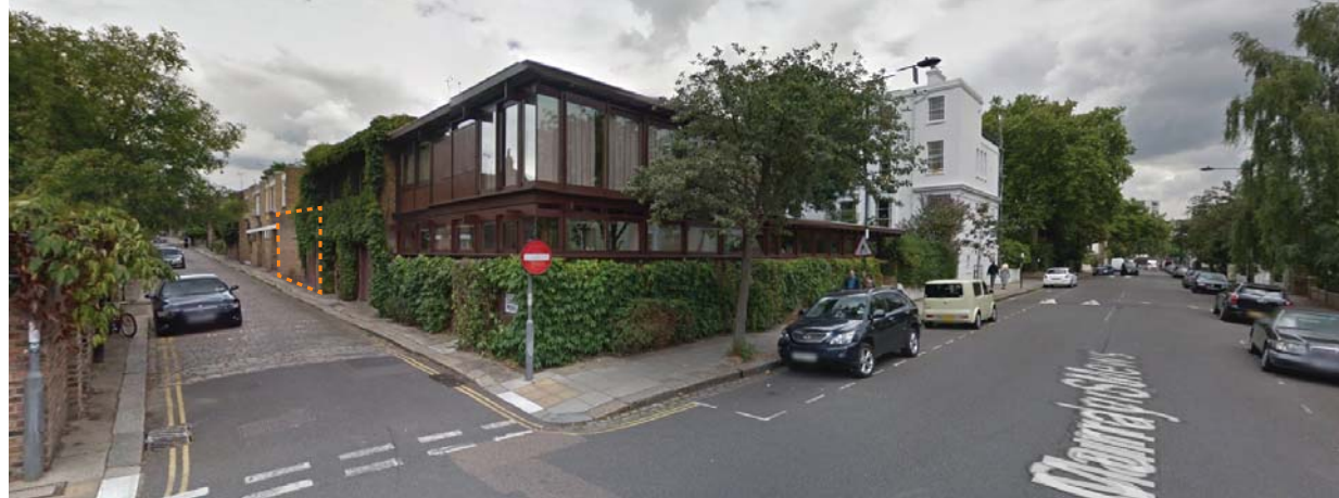
Figure 3. View of Camden Mews from Murray Street, looking east. The modern corner building was noted as exemplary by the Camden Square Conservation Area Appraisal and Management Strategy. Existing wall highlighted
