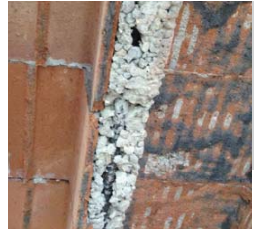
Honeycombing of concrete beams
