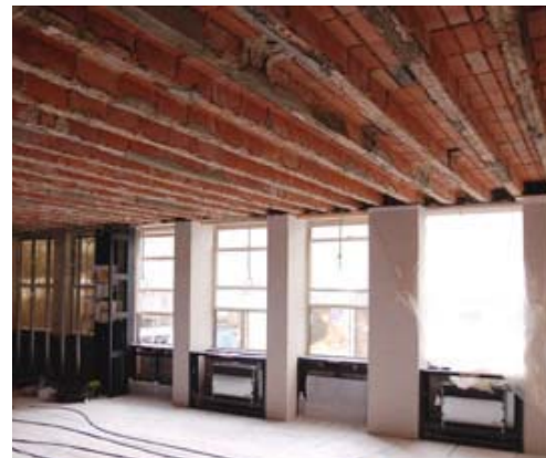
Existing structure following plaster and tile removal
