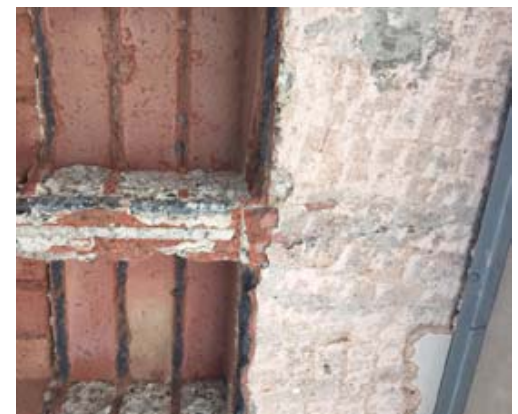
Honeycombing of concrete beams
