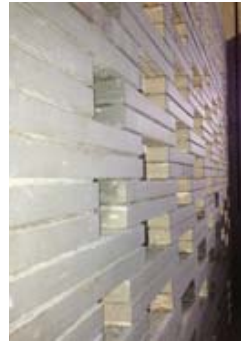
Brick weave appears solid especially from oblique angles
