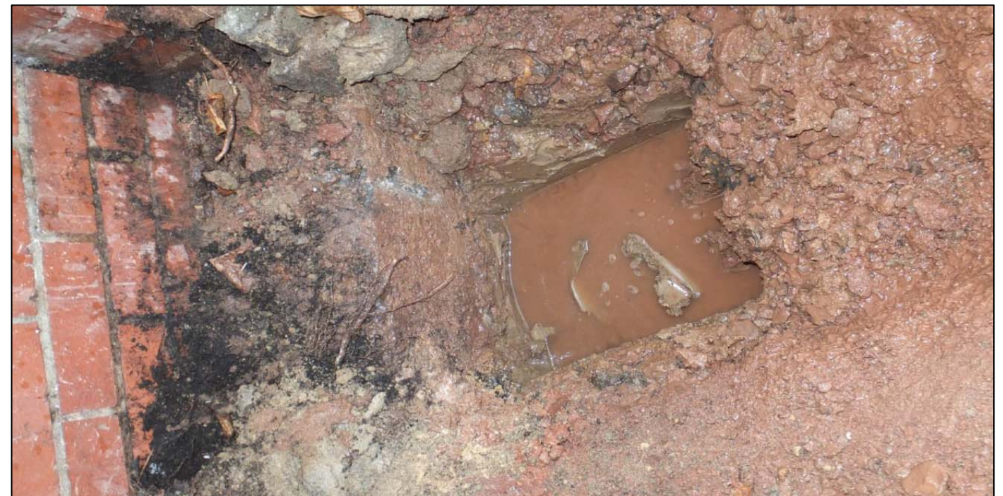
Figure 8: Trial Pit Undertaken to Confirm the Existing Eastern Boundary Condition
