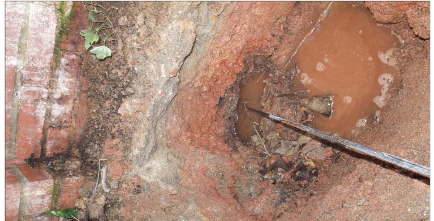
Figure 7: Trial Pit Undertaken to Confirm the Existing Western Boundary Condition
