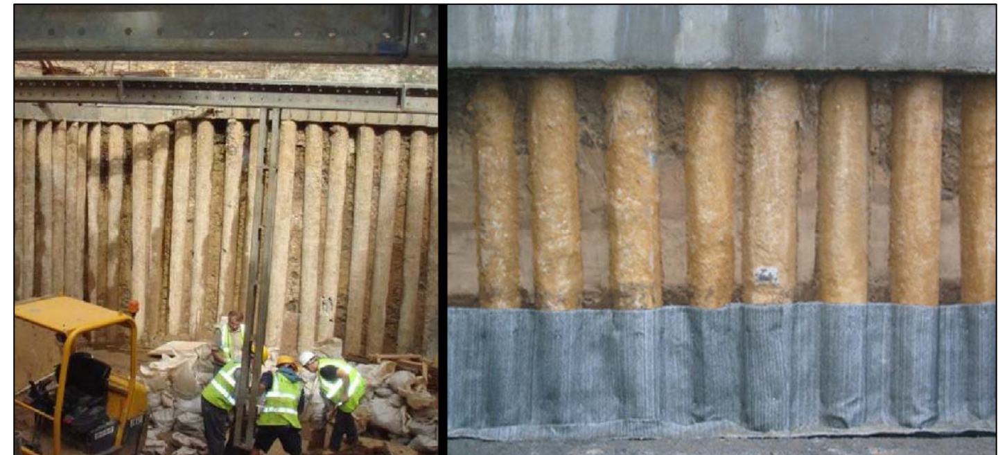
Figure 11: Propped Contiguous Pile Construction
