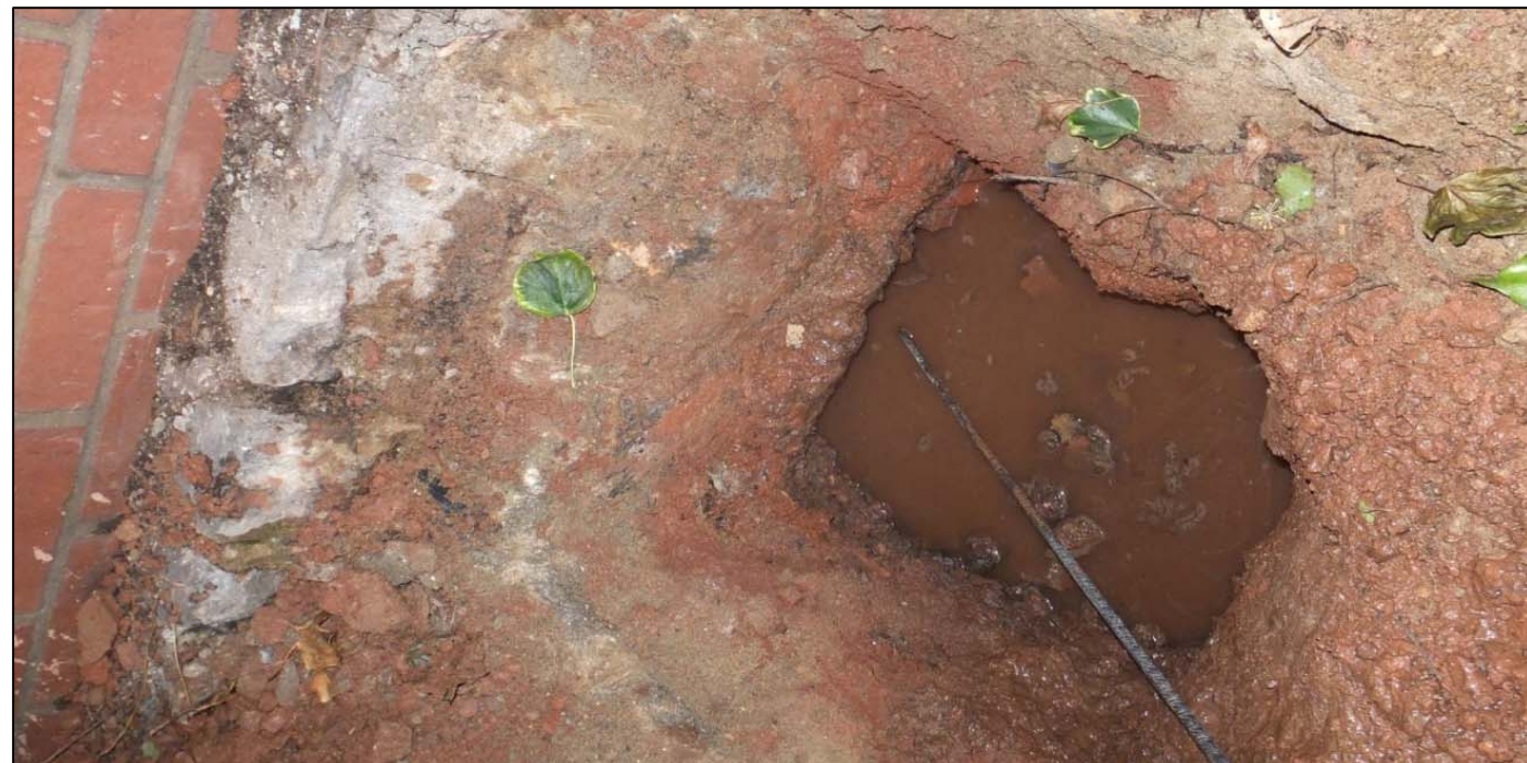
Figure 6: Trial Pit Undertaken to Confirm the Existing Northern Boundary Condition
