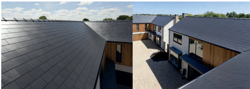
Private House Barnoldby Road (Grimsby, England)
