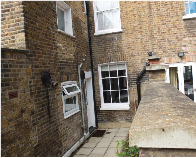
Rear garden of no.11 looking over boundary wall with no.9
