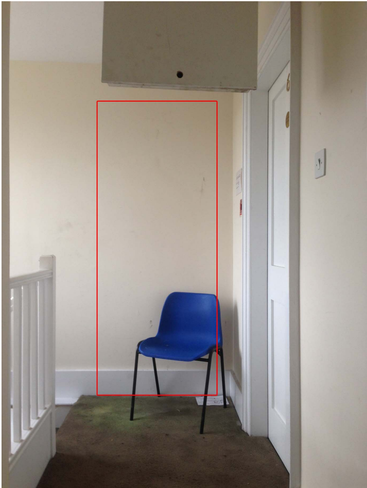
Above: location of new door opening up.
