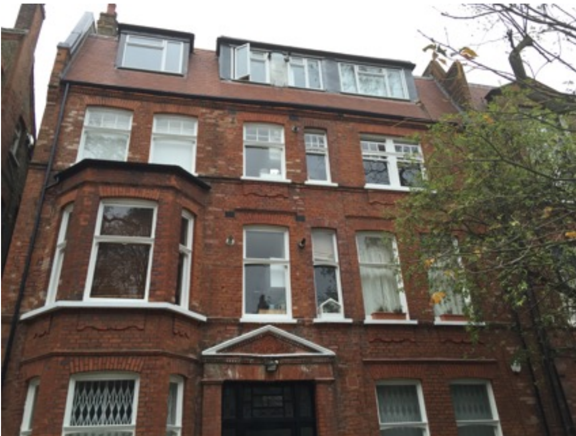
Example of dormer to neighbour at 112, not part of the the original build.
