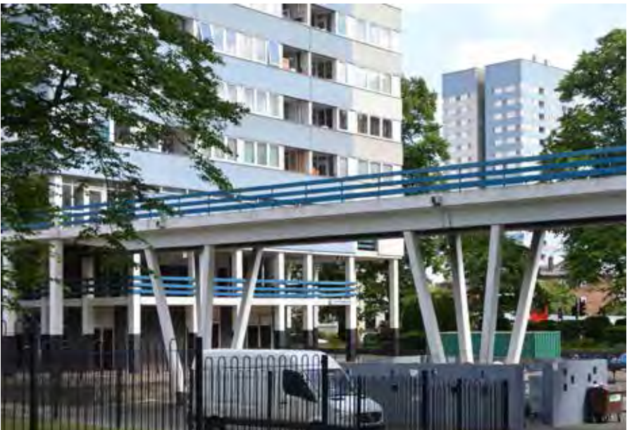
Existing space between the towers
