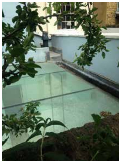
IMAGE 2.17. CONSERVATORY ROOF VIEWED FROM SHED ROOF
