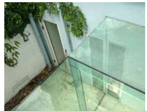
IMAGE 2.13. CONSERVATORY ROOF + SIDE KITCHEN DOOR
