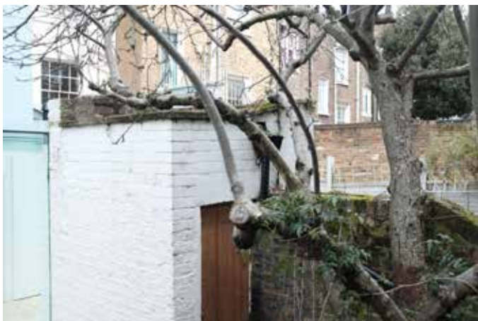
IMAGE 2.19. SHED AND BOUNDARY WALL JUNCTION
