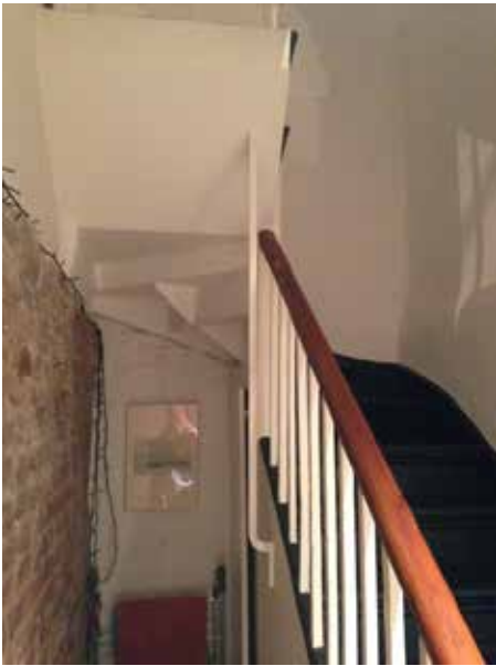
IMAGE 8.1. LOWER GROUND FLOOR STAIRCASE + BALLUSTRADE
