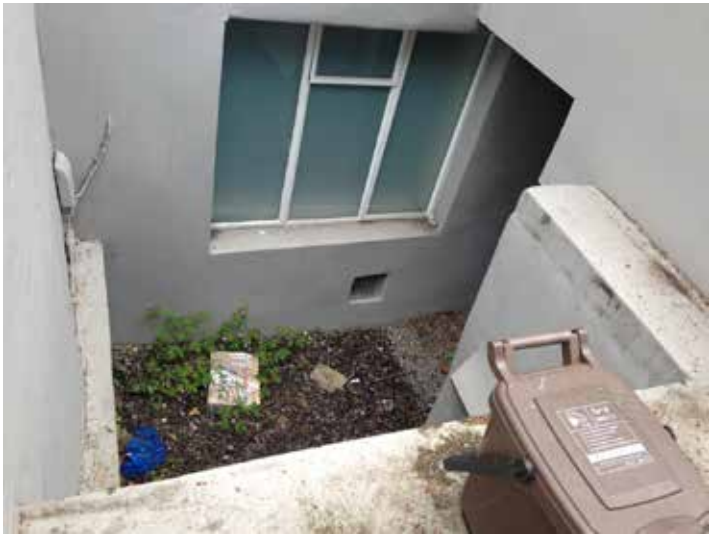
IMAGE 3.1. BASEMENT FRONT FACADE WINDOW
