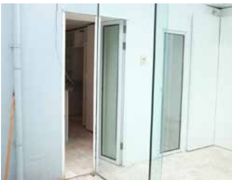
IMAGE 2.8. REAR KITCHEN DOORS TO GARDEN + CONSERVATORY
