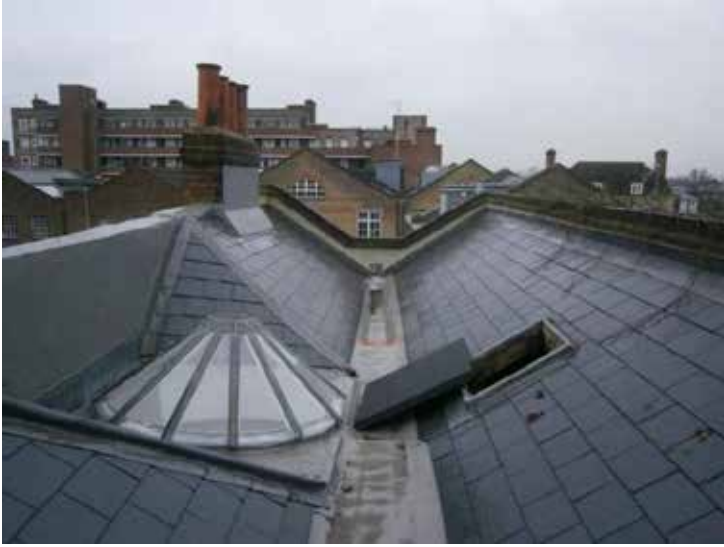
IMAGE 9.1. ROOF LOOKING SOUTH
