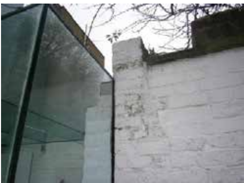
IMAGE 2.11. DETAIL GLAZED JUNCTION WITH SHED
