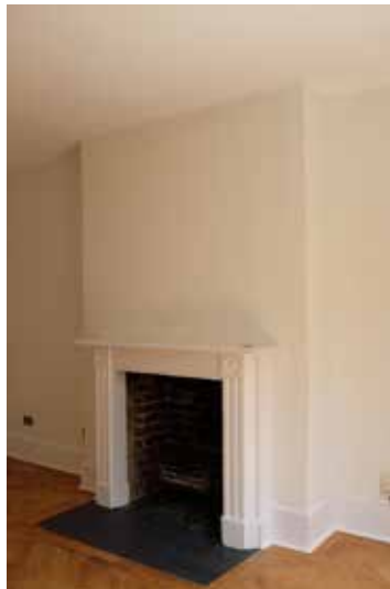
IMAGE 5.7. FIREPLACE + SKIRTING TO BE RETAINED
