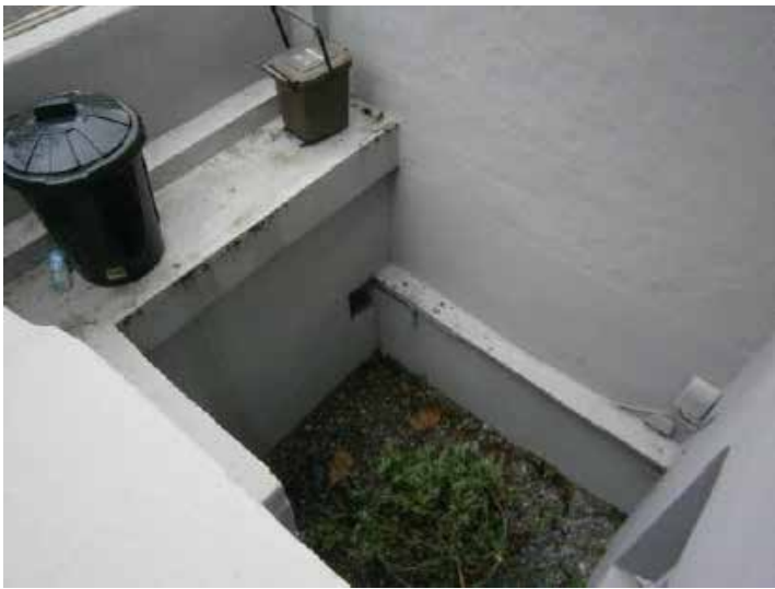
IMAGE 3.3. BASEMENT LIGHTWELL FRONT WALL
