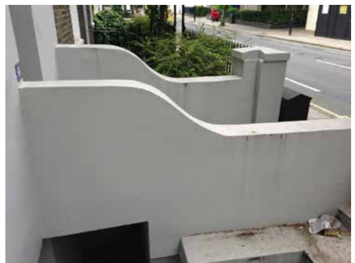
IMAGE 3.4. ENTRANCE STAIRWAY WALL
