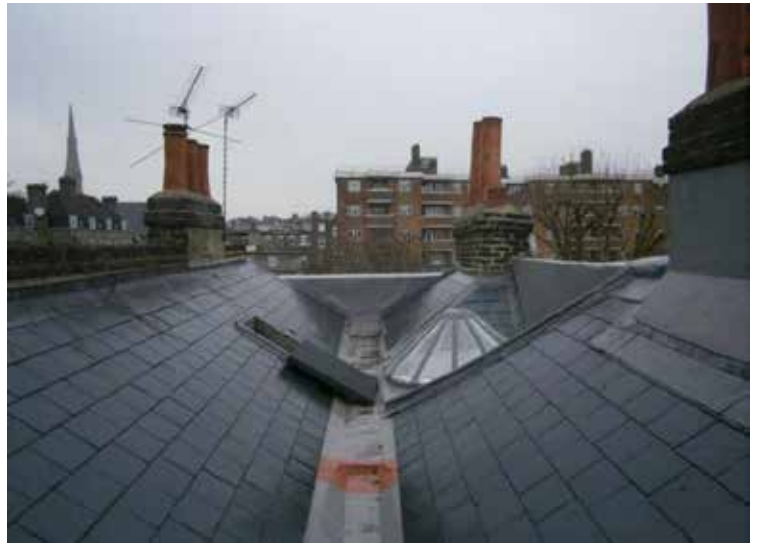
IMAGE 9.2. ROOF LOOKING NORTH
