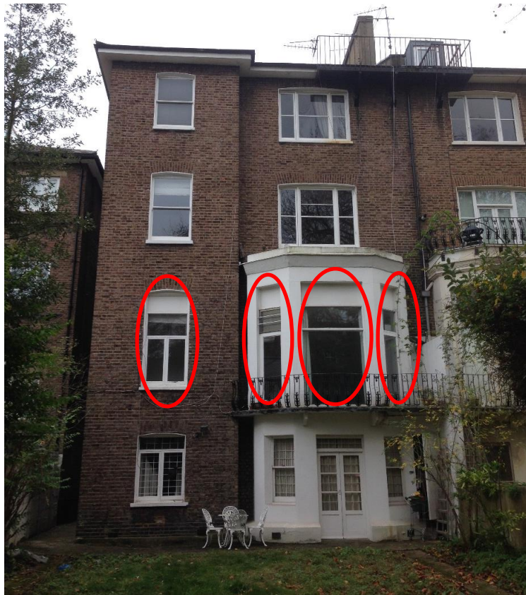
Figure 1 – Rear elevation and the windows marked for replacement (red)
