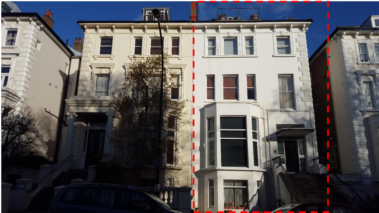
Front elevation of the above addressed property (marked in red)
