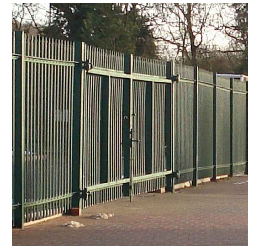
2. Proposed 1m width x 2.4m high Barkers ProtectorGate single leaf pedestrian gate. Type and finish to match existing as shown in image 1.
