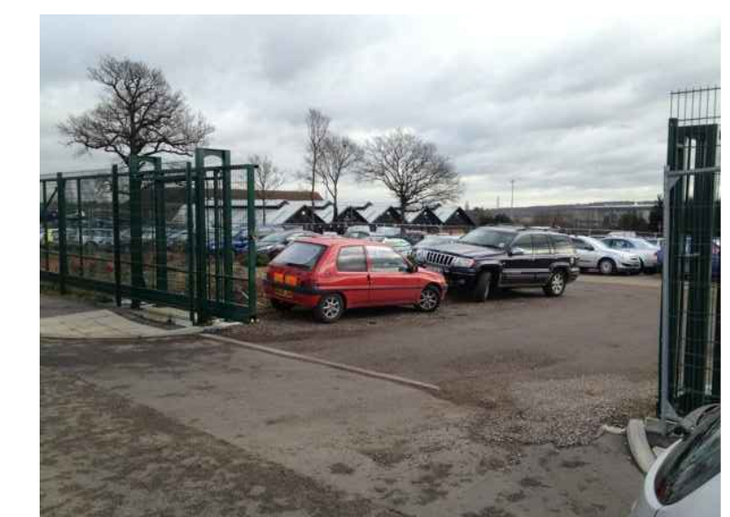
1. Proposed 4m high x 12m wide manual sliding gate to match fence type 358. Finish to match existing.
