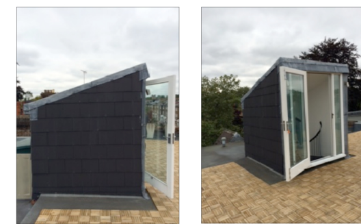
PHOTOS SHOWING EXISTING STAIRCASE & ENCLOSURE
