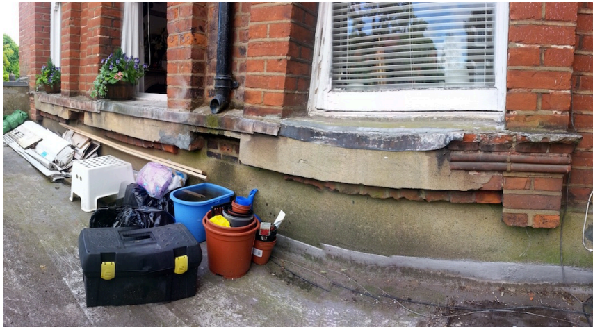
Brickwork under windows already removed - unaesthetic finish
