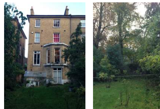
Rear view of property and of garden
