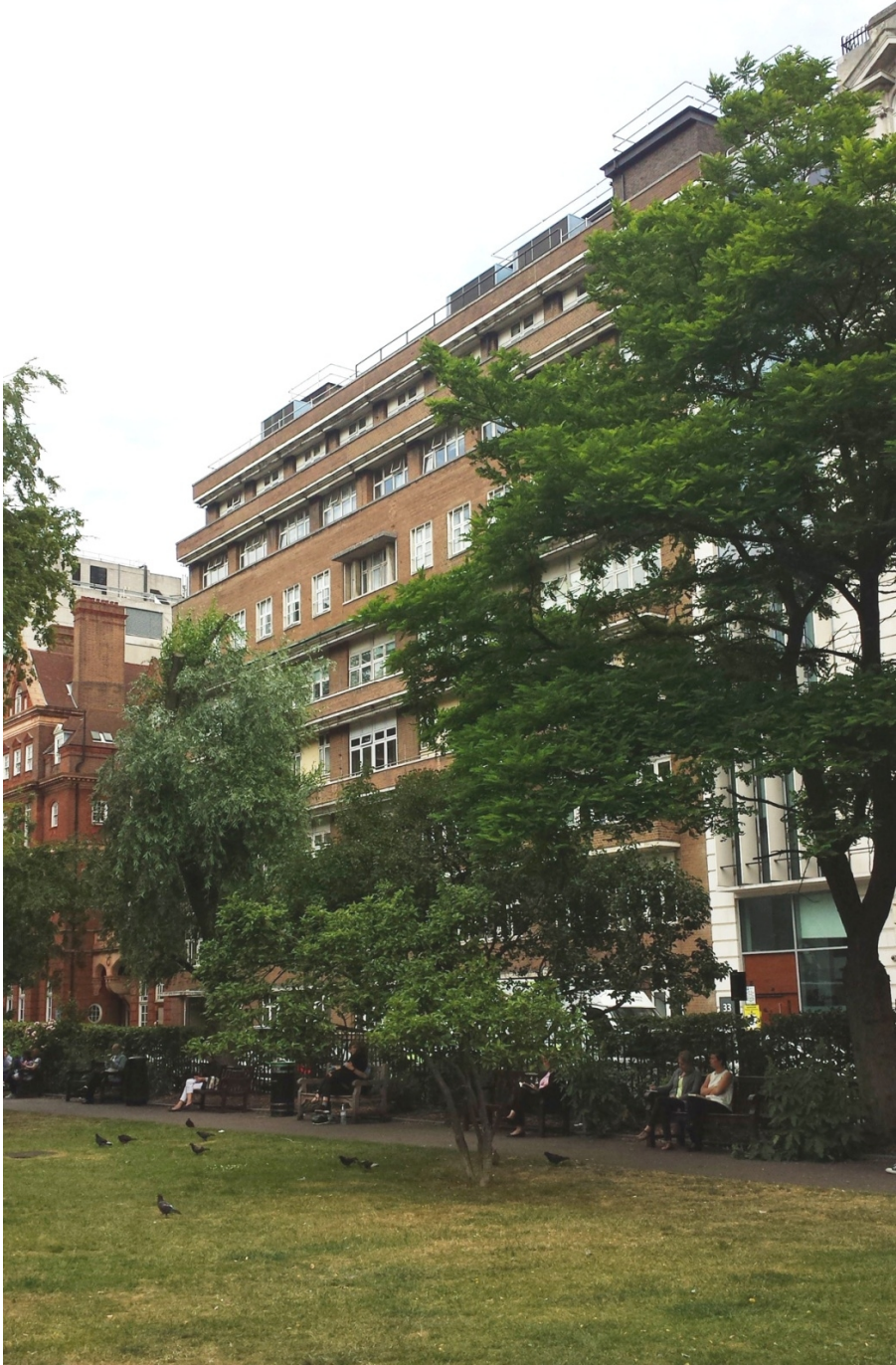
Queen Mary Wing, view from Queen Square Existing roof plant - partially visible at 8 th Floor, behind the low parapet wall
