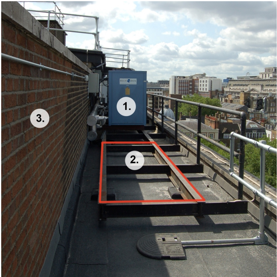
Roof terrace, southwest (Queen Square side), 8 th floor, Queen Mary Wing
