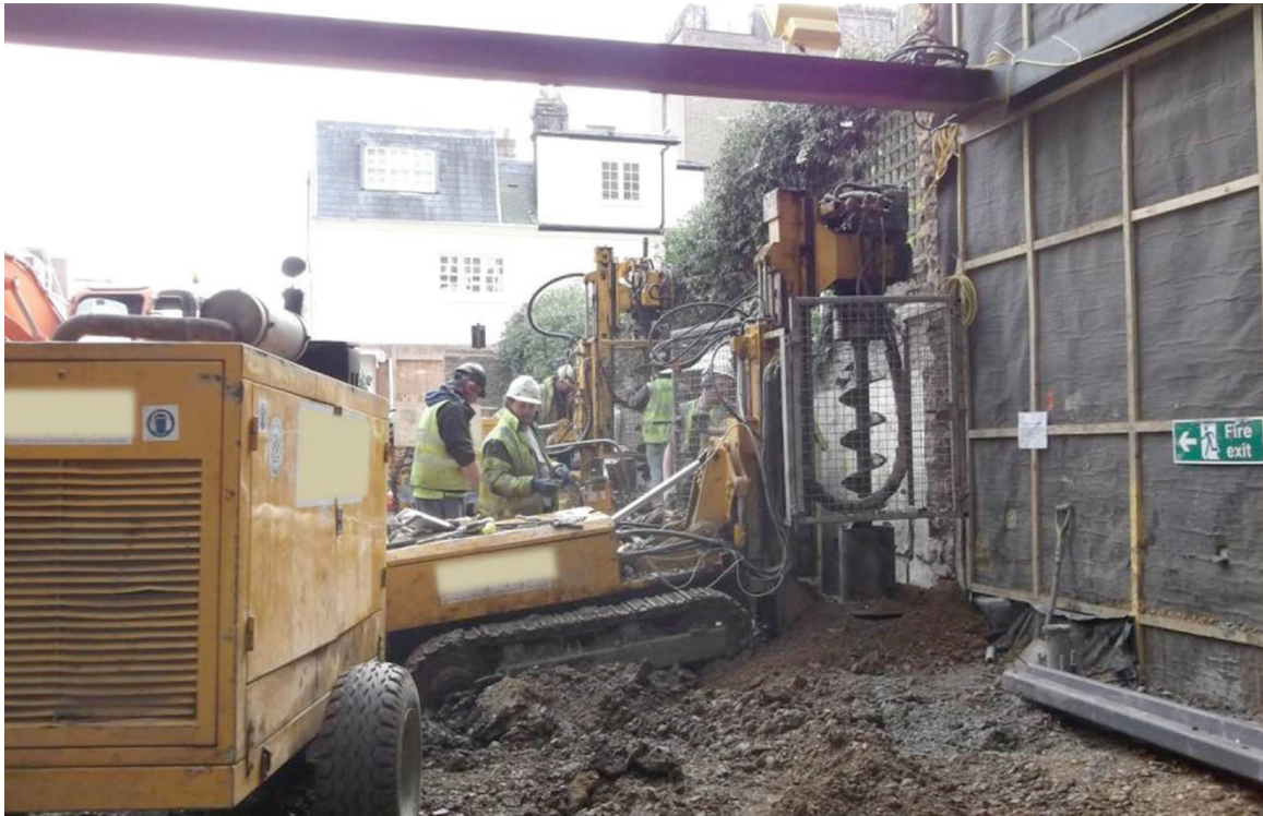
Figure 4 Piling rig at work within basement
