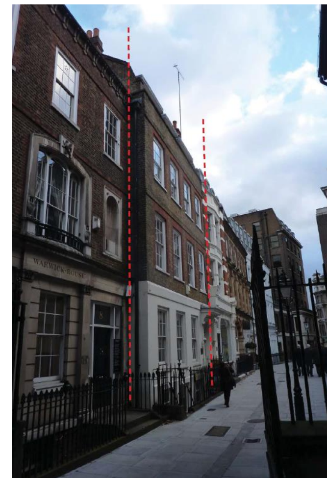
Existing Front Elevation of 7 Warwick Court
