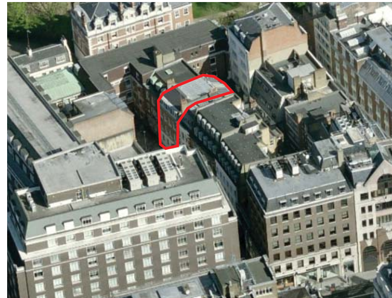
Warwick Court and Surroundings Aerial View 01 (Site outlined in red)
