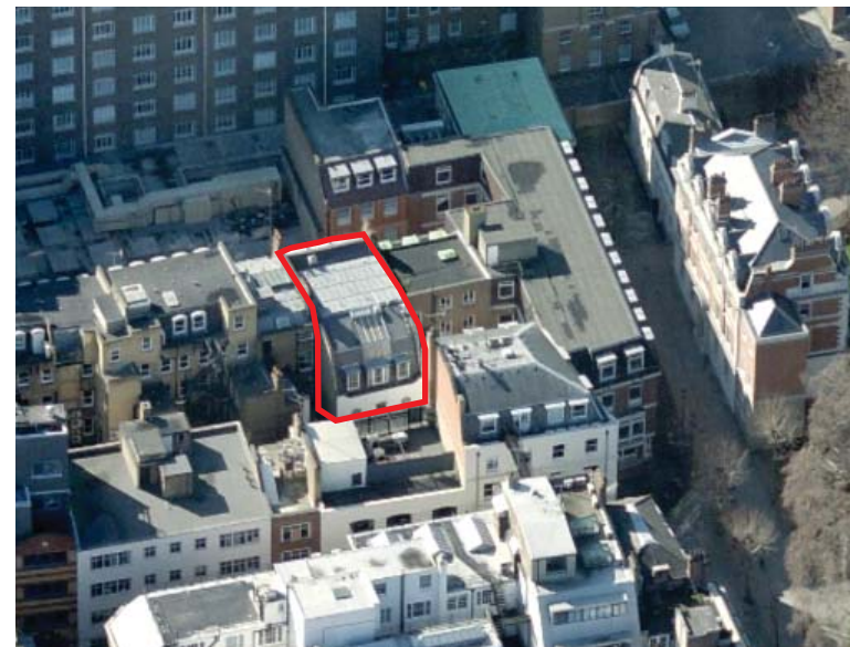
Warwick Court and Surroundings Aerial View 02 (Site outlined in red)
