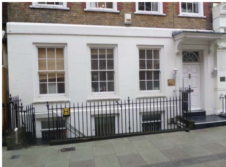
Fig. 2/ 7 Warwick Court front elevation (showing ground and part of the lower ground floors).
