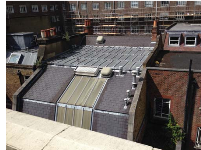
7 Warwick Court Rear extension roof
