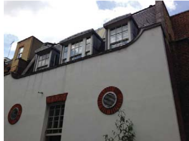
7 Warwick Court Rear elevation
