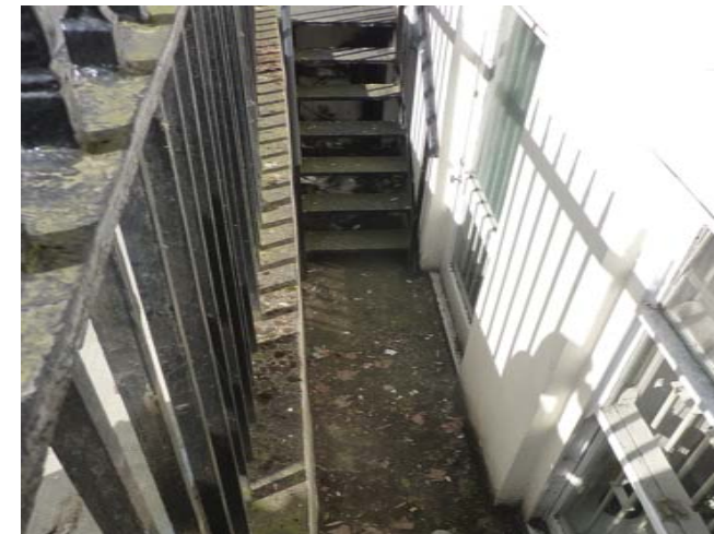
7 Warwick Court Front Lightwell
