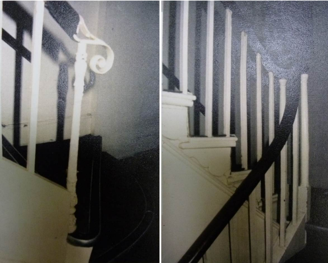
Fig. 33 Record photos of staircase, 1990 (left: ground floor newel post, right: landing between ground and first floors) (LB Camden, planning file)
