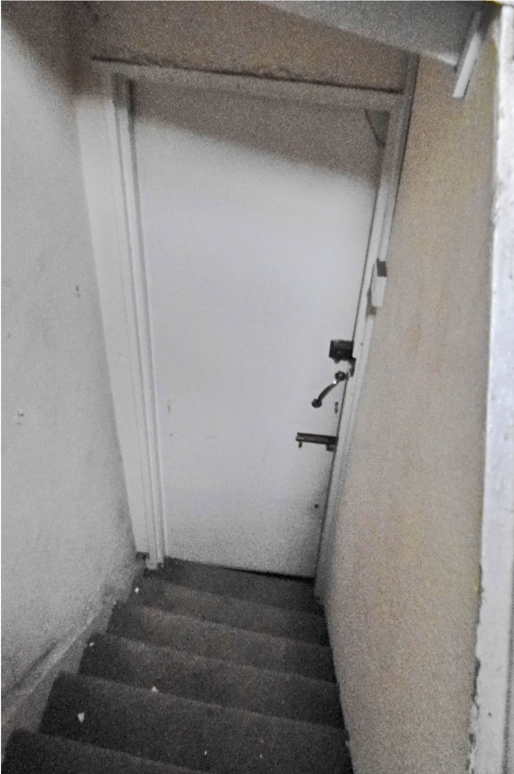
Existing flat entrance door, viewed from flat internal stair landing
