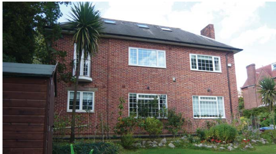
VIEW 3 - No.6 VIEW FROM REAR GARDEN
