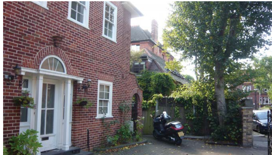
VIEW 2 - No.6 FRONT ENTRANCE
