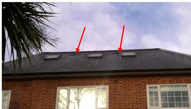
**Plate 4.3: Missing and slipped tiles of southern elevation.**
