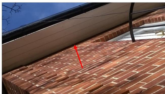
**Plate 4.3: Gap between soffit and brickwork.**
