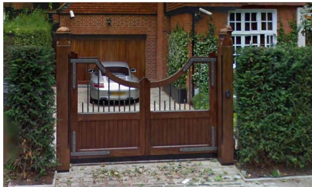
Figure 4.3.1: Existing fence at 11 Wadham Gardens
