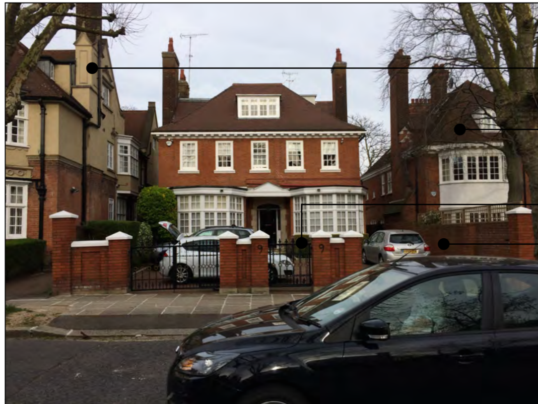
Figure 3.2.1: Front facade seen from Harley Road
