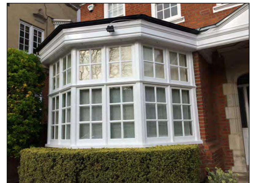
Figure 3.2.5: Front facade window bay
