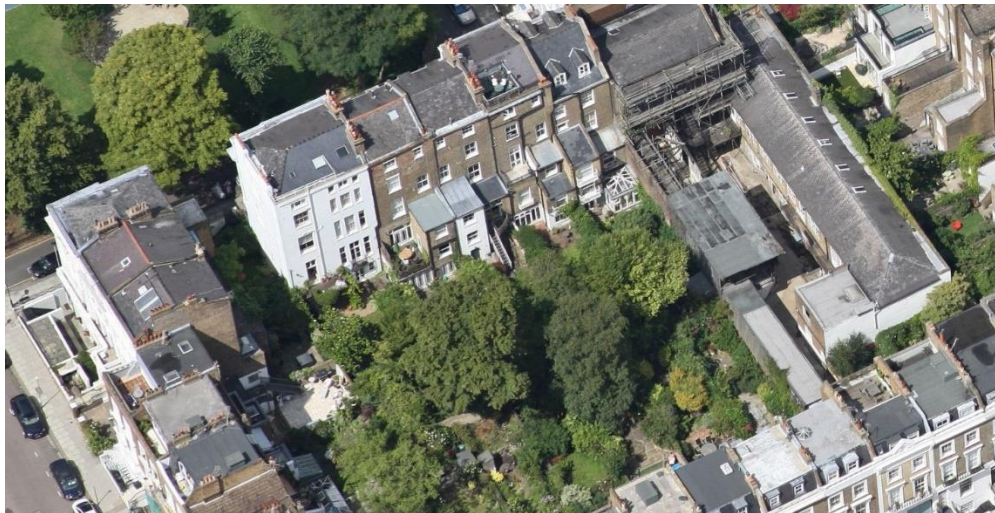
AERIAL VIEW WEST – to Chalcot Square
