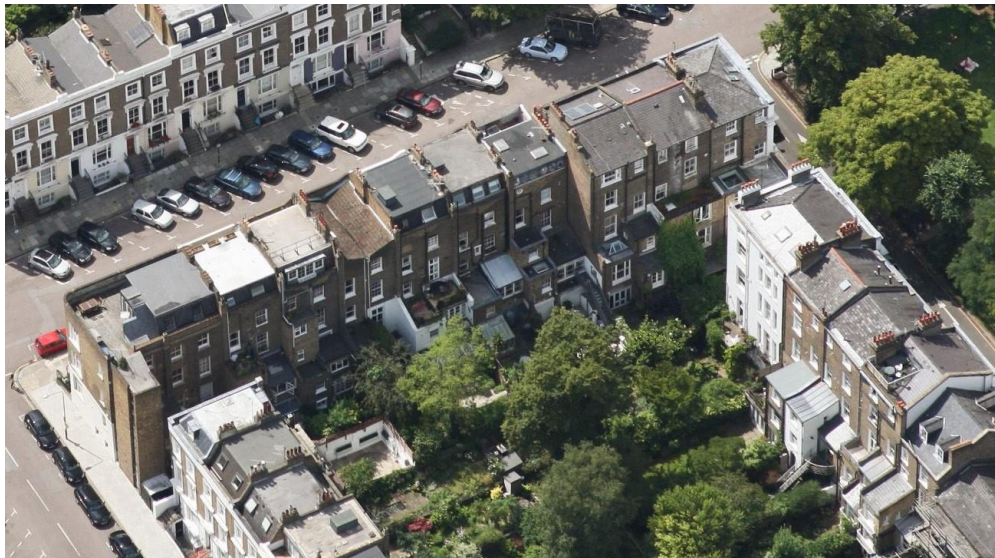
AERIAL VIEW SOUTH – to Chalcot Road
