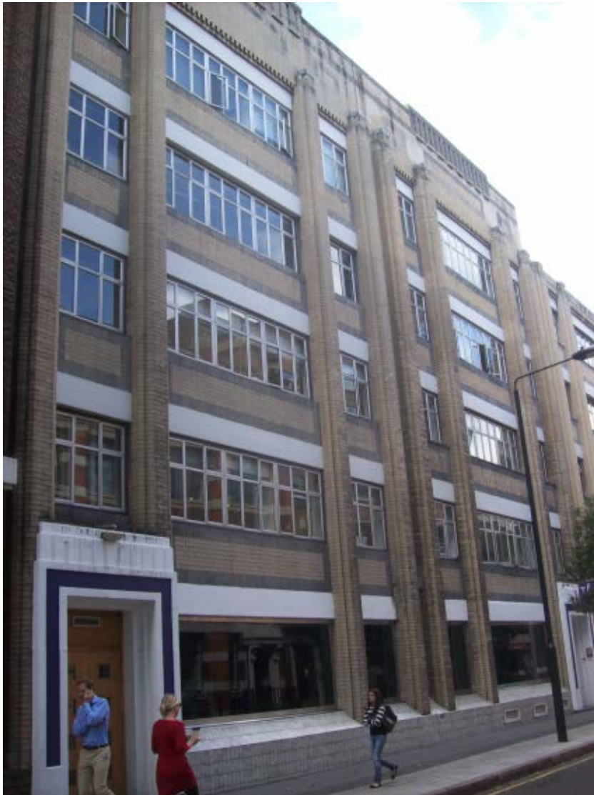
Figure 2 - 71-81 Whitfield Street existing façade
