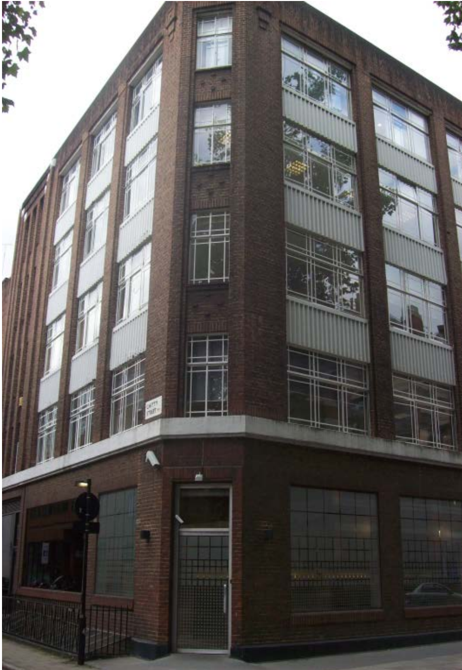
Figure 7 - 67-69 Whitfield Street existing façade
