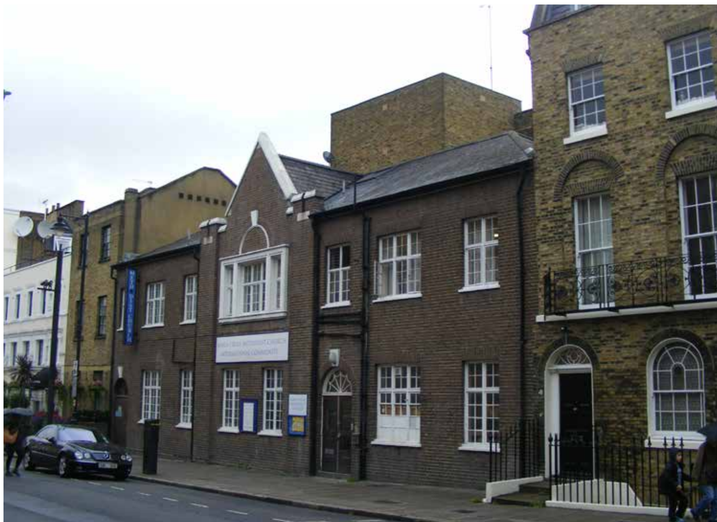
Existing frontage to Crestfield Street
