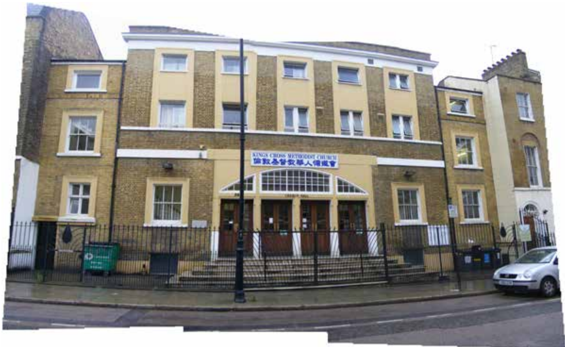
Existing, adapted frontage to Birkenhead Street
