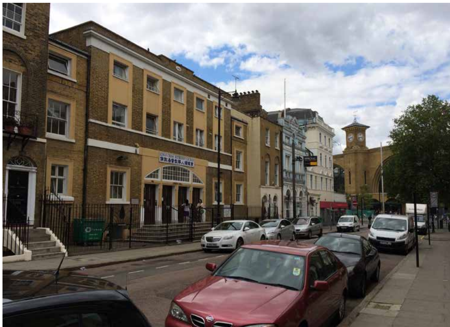
Existing frontage to Birkenhead Street
