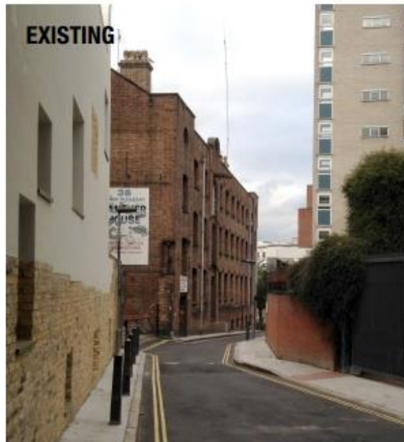
Existing condition of Panther House
