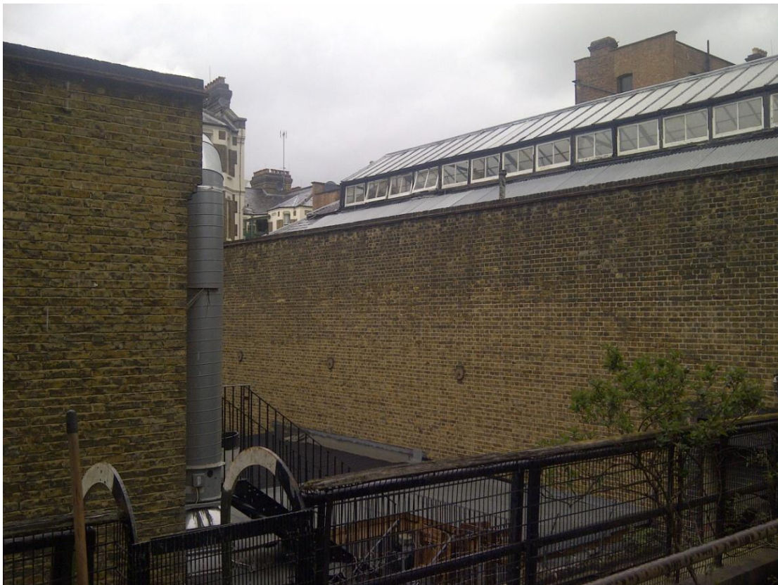
The Brain Yard building (glazed roof) as viewed from the rear of 156 Gray's Inn Road and with the rear of 160 Gray's Inn Road visible on the left of the image
