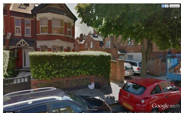
Side of Building – Louvres at high level on Ground Floor
