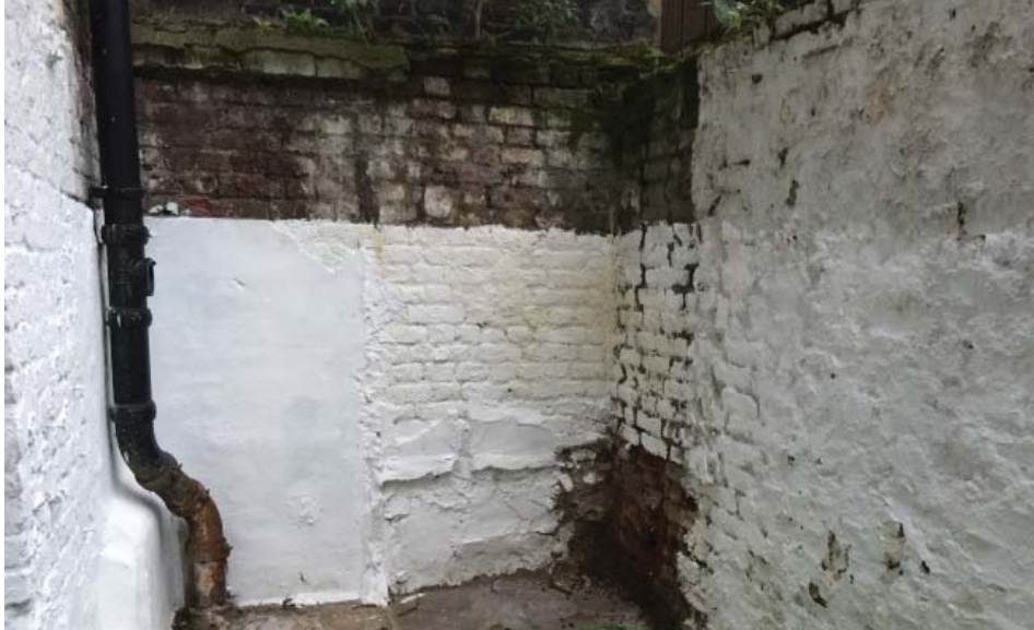
fig 6. view into existing rear courtyard
