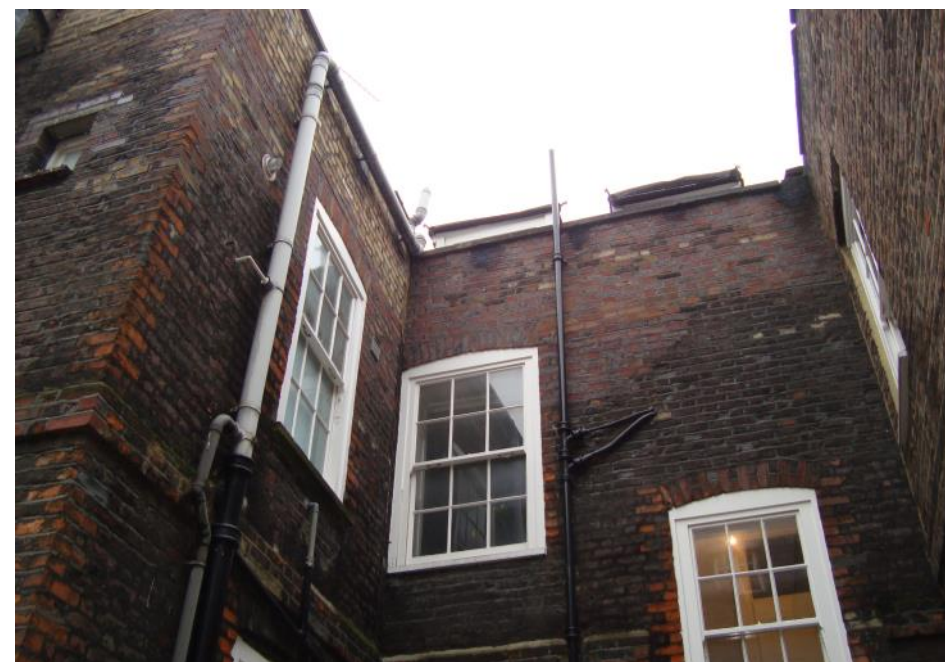
Figure 18: Rear elevation of 35 Great Queen Street, showing some rebuilding at the upper levels, using yellow brick. Photograph taken from the roof of the flat roofed rear extension.
