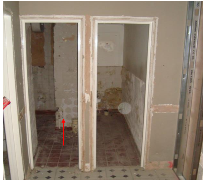
Figure 32: The spur of wall seen through the left hand doorway would be removed to allow reconfiguration of the bathroom facilities. These works are confined to the later extension of the basement, outside of the original basement area, and would not affect any historic fabric from the original property.
