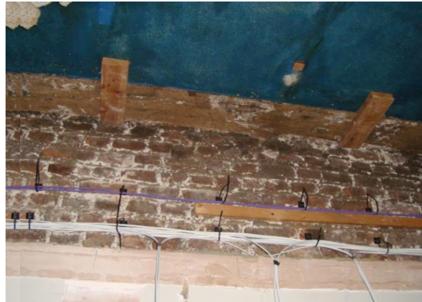
Figure 30: Brickwork to be cleaned and left exposed, with plasterboard seen beneath to be removed.
