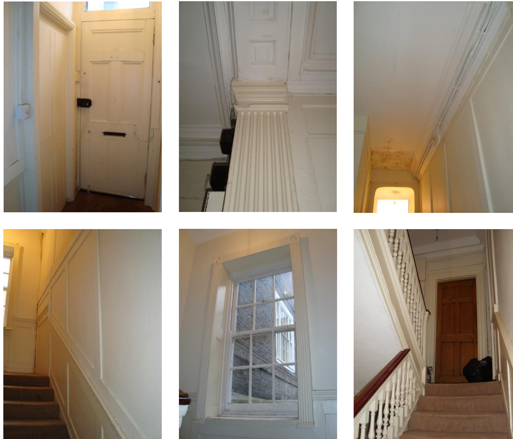
Figure 25: Photographs of surviving features of architectural interest in communal areas, including (clockwise from top left): lobby space with blocked original door, fluted pilaster in the hallway, cornice detailing in hallway, nineteenth century staircase and landing area, decorative window surround on half landing and plain panelling on the staircase.
