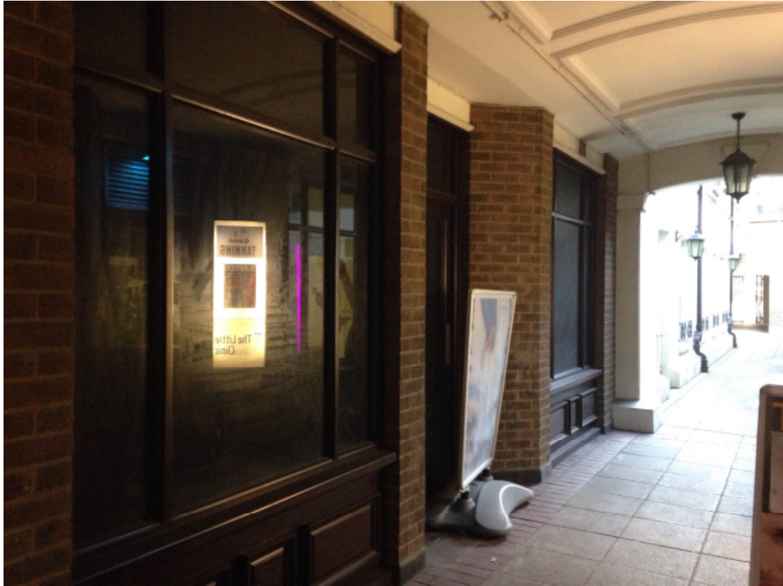
Vacant shop unit within the pedestrian accessway
