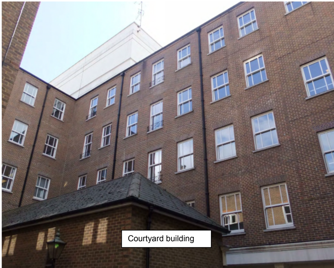
Eastern rear elevation of no. 2 – 8 Bloomsbury Street
