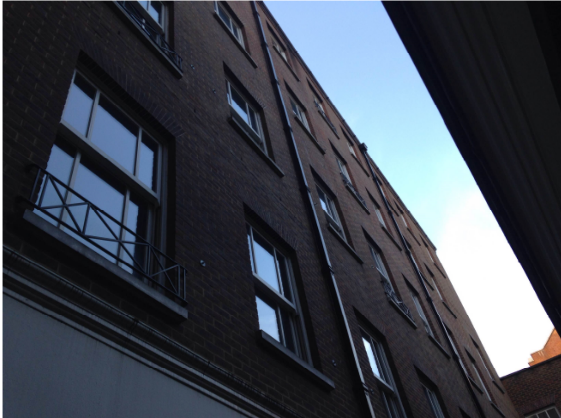
View of the rear eastern elevation of no. 2 – 8 Bloomsbury Street
