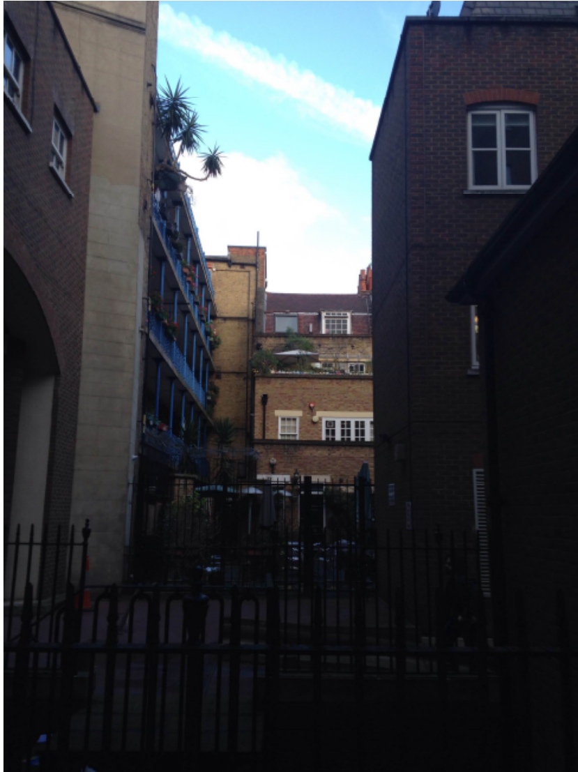
View of rear elevation of residential flats at no. 3 Stedham Place from the pedestrian accessway between New Oxford Street and Streatam Street
