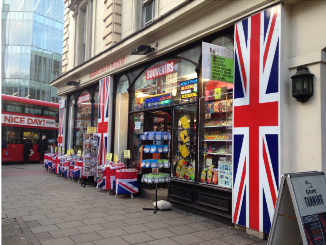
No. 52-56 New Oxford Street ground floor shopfront
