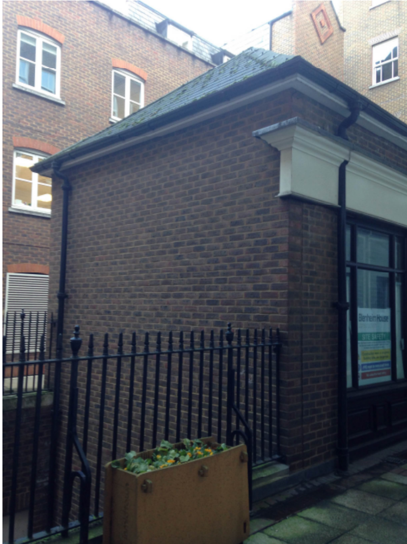
Rear elevation of single storey courtyard building fronting the pedestrian accessway from New Oxford Street to Streatham Street
