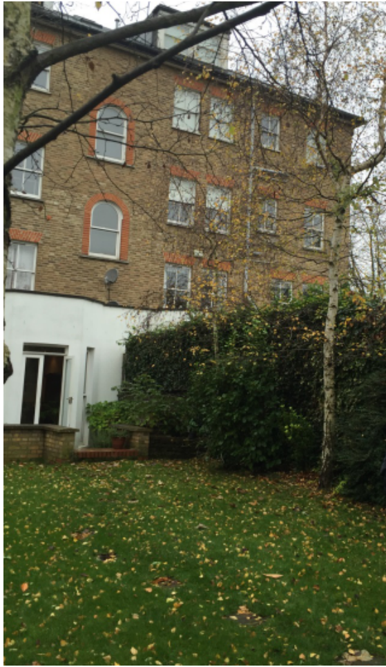
Photo 5 – View back to dwelling property
