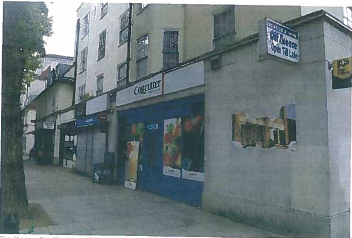
The Phoenix Road frontage of the two shops, showing the projecting signs, modern shopfronts, and upper fascias. Note also how the original doorway in the wall on the right has been completely blocked.
