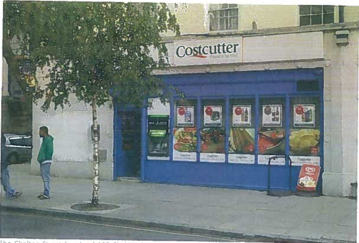
The Chalton Street façade of 100 Chalton Street, showing the modern shopfront and upper fascia, and the cashpoint by the door
