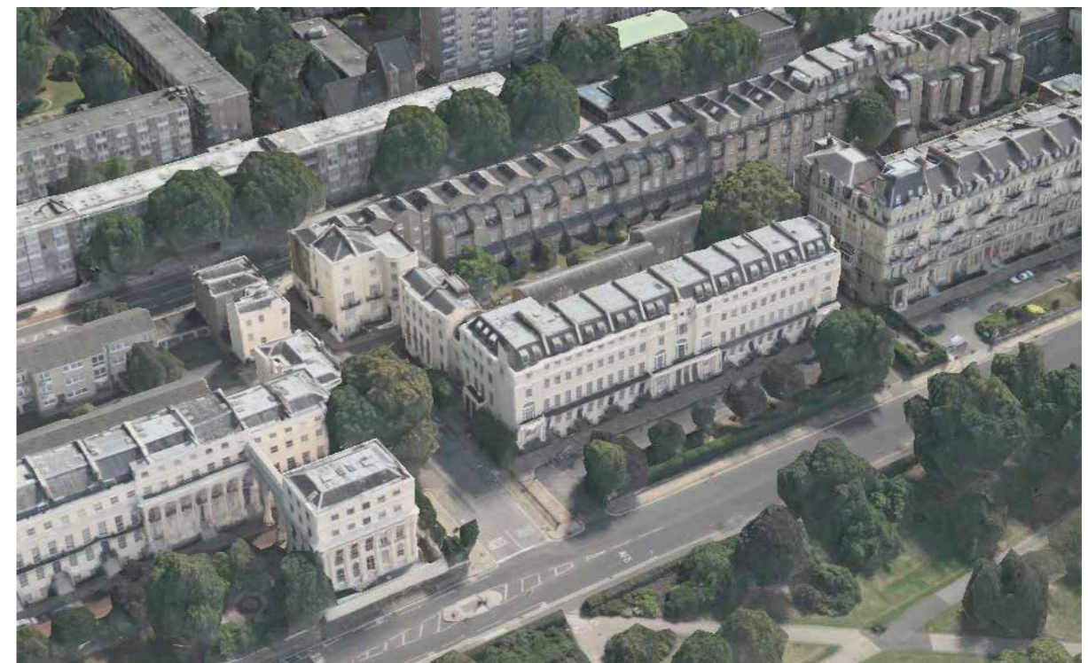
Aerial view showing corner of Cambridge Terrace and Chester Gate
