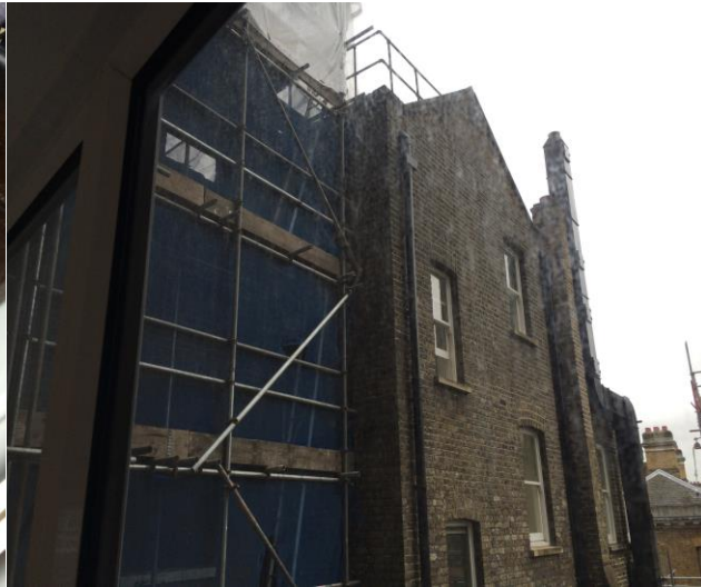
Flue on neighbouring building
