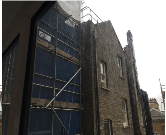
Flue on neighbouring building
