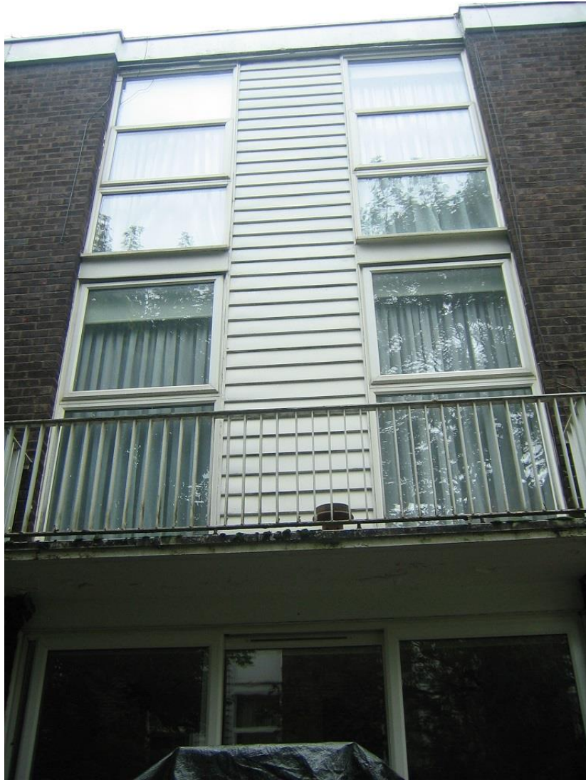
Photo 3- Rear Elevation Upper Floors
