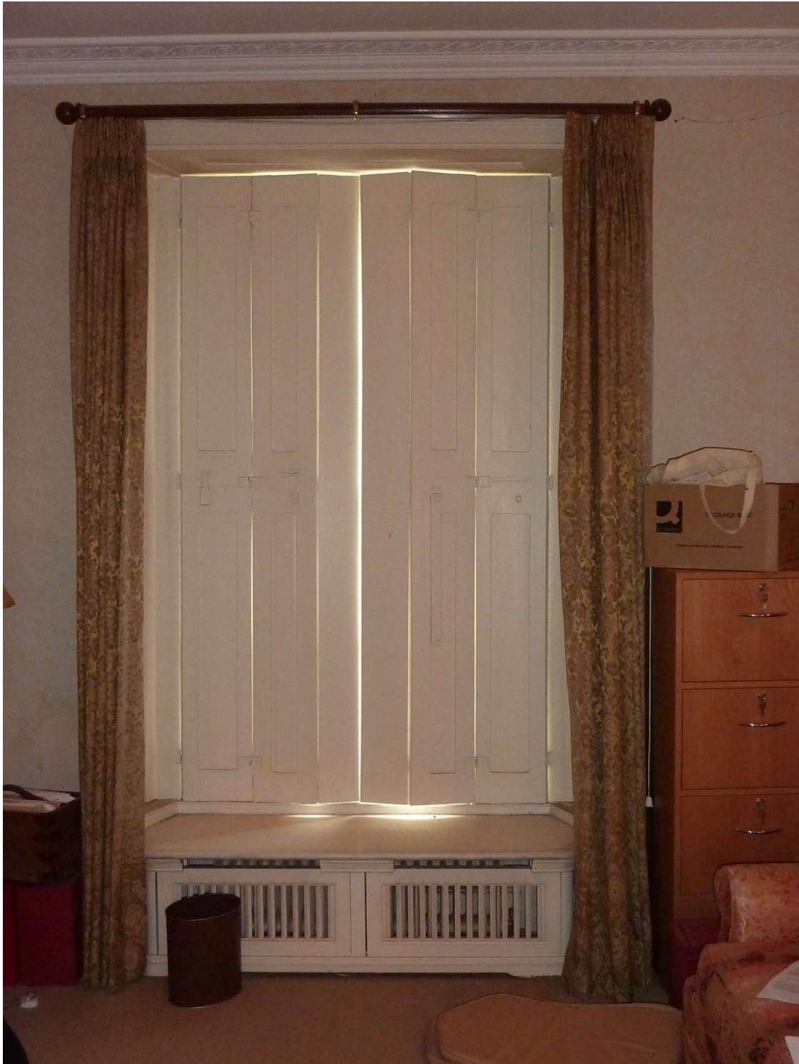
Fig 1: Image of upper ground floor existing shutter, (which the new / proposed first floor shutters are based upon).
