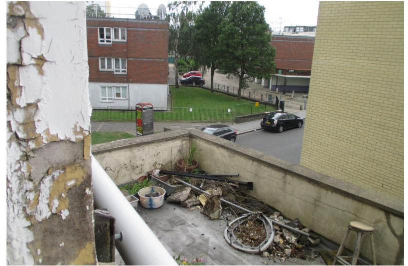
1.5 Side of site looking at QC
