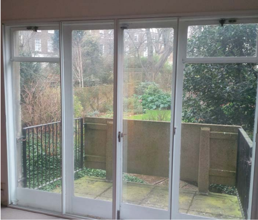
1. ALUMINIUM FRAME SECONDARY GLAZING (D.06)
