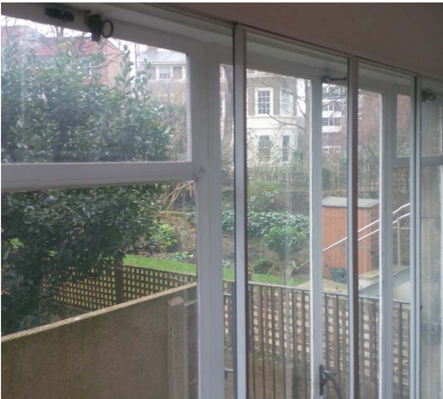
2. ALUMINIUM FRAME SECONDARY GLAZING (D.06)
