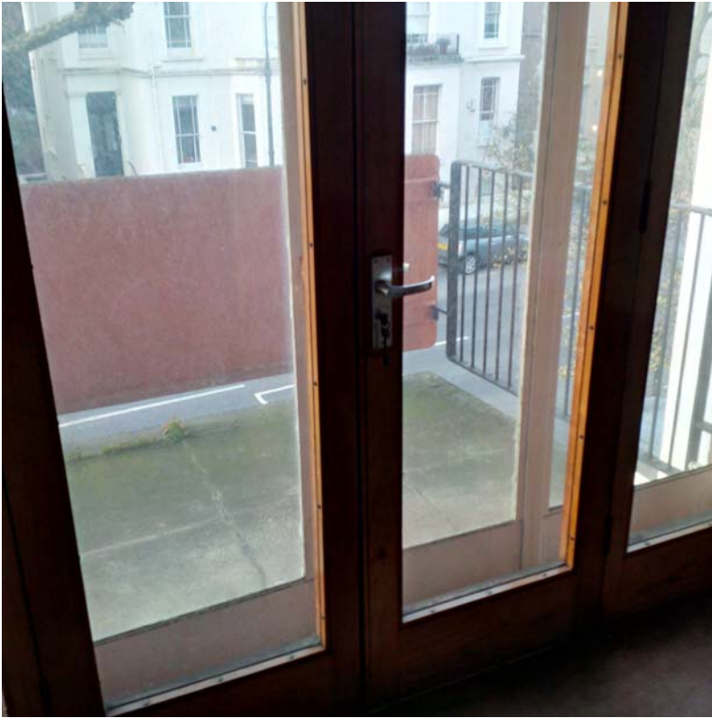
7. FLAT E - WOODEN FRAME SECONDARY GLAZING
