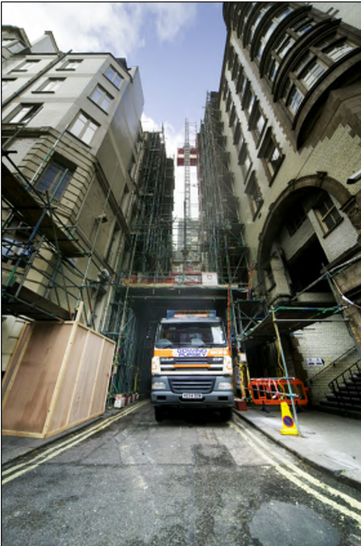
PHOTO 1: THE SAVOY HOTEL DURING CONSTRUCTION
