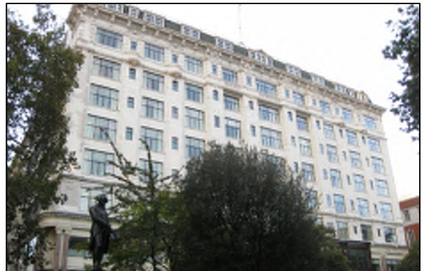
PHOTO 3: THE SAVOY HOTEL POST CONSTRUCTION
