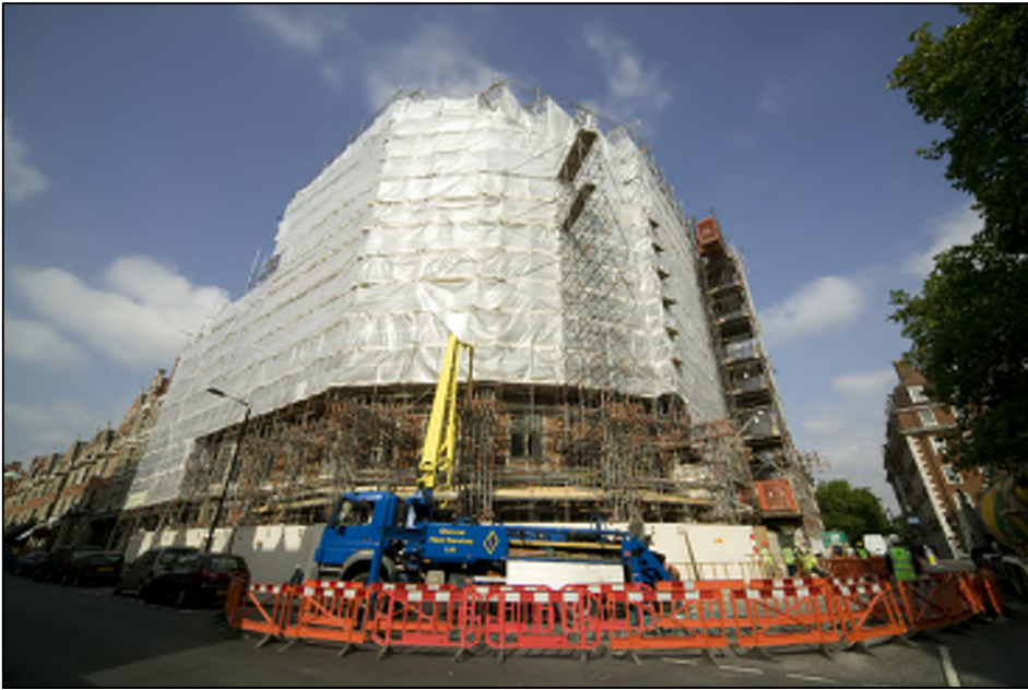
PHOTO 1: THE CONNAUGHT HOTEL DURING CONSTRUCTION
