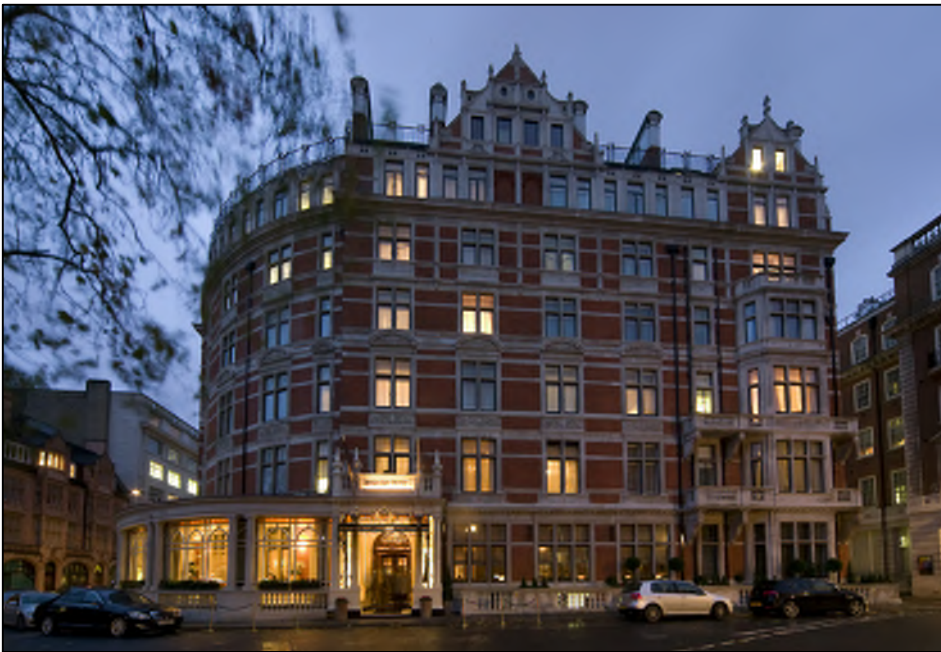
PHOTO 2: THE CONNAUGHT HOTEL POST COMPLETION
