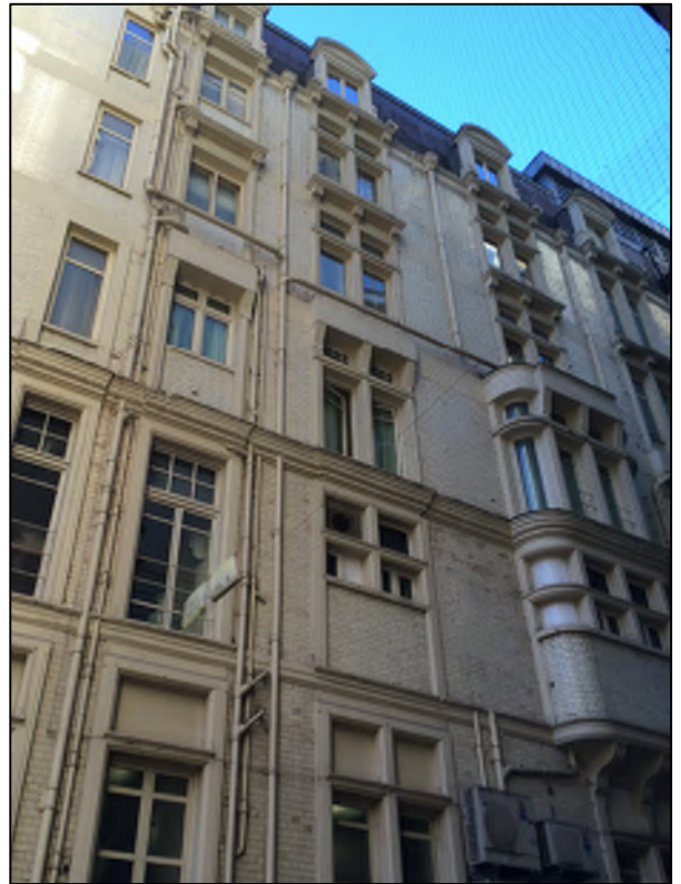
PHOTO 2: THE SAVOY HOTEL POST CONSTRUCTION (AREA OF HOIST)
