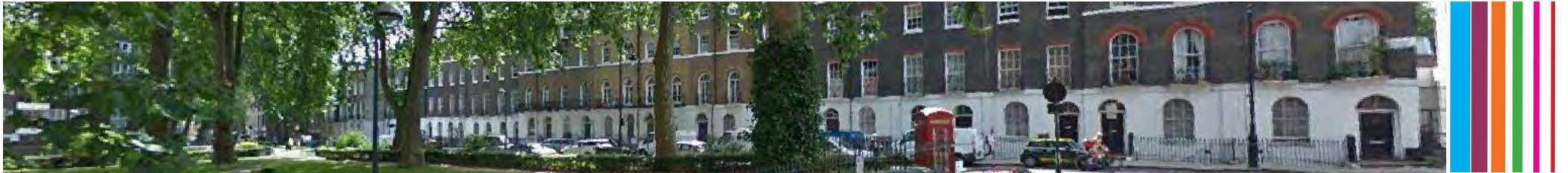
No. 5 Regent Square - Window Repairs & Refurbishment
