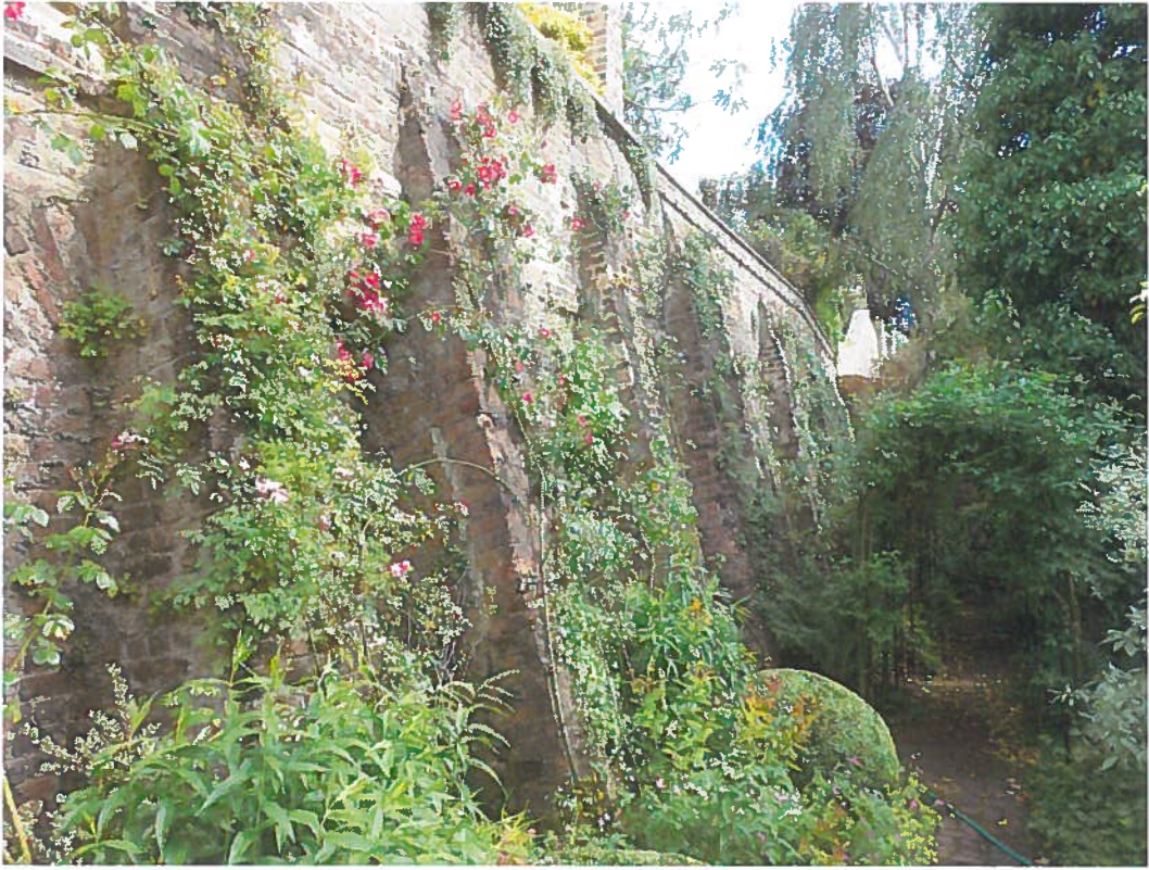
Photo 33 – Retaining wall to upper garden
