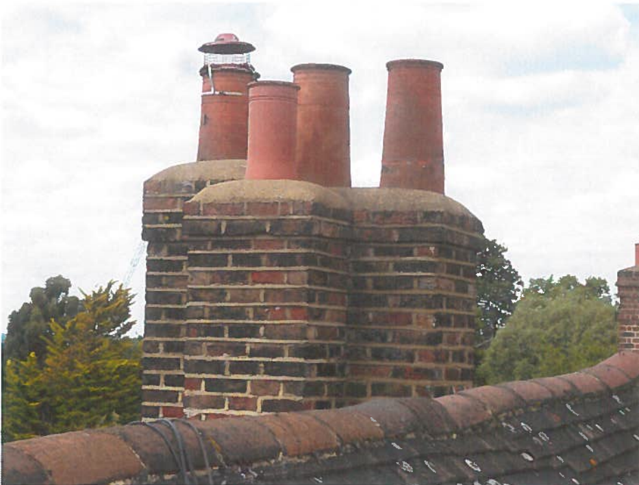
Photo 2 – North west chimney
