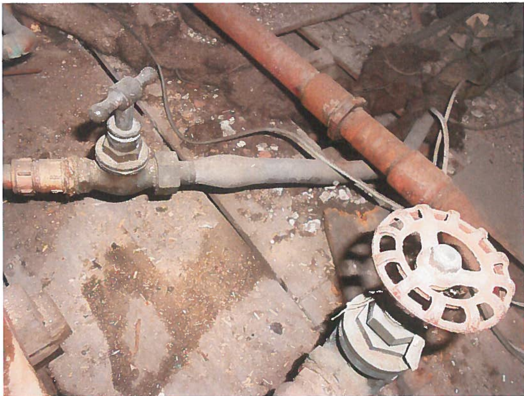
Photo 28 – Lead and iron piping in roof space
