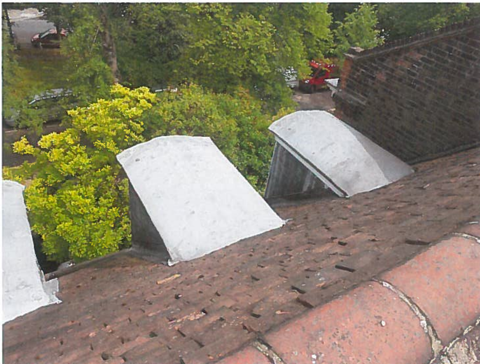
Photo 4 – Main roof – front slope
