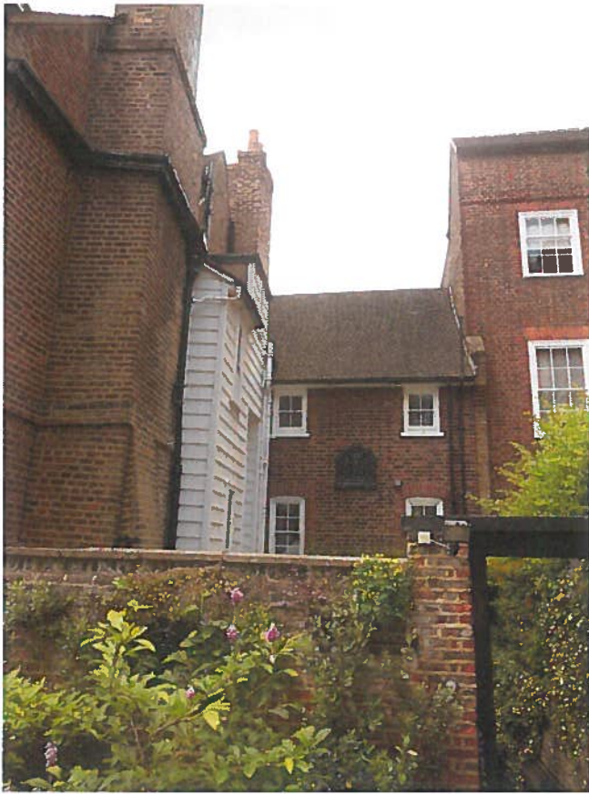
Photo 15 – Front elevation (north extension and annexe)
