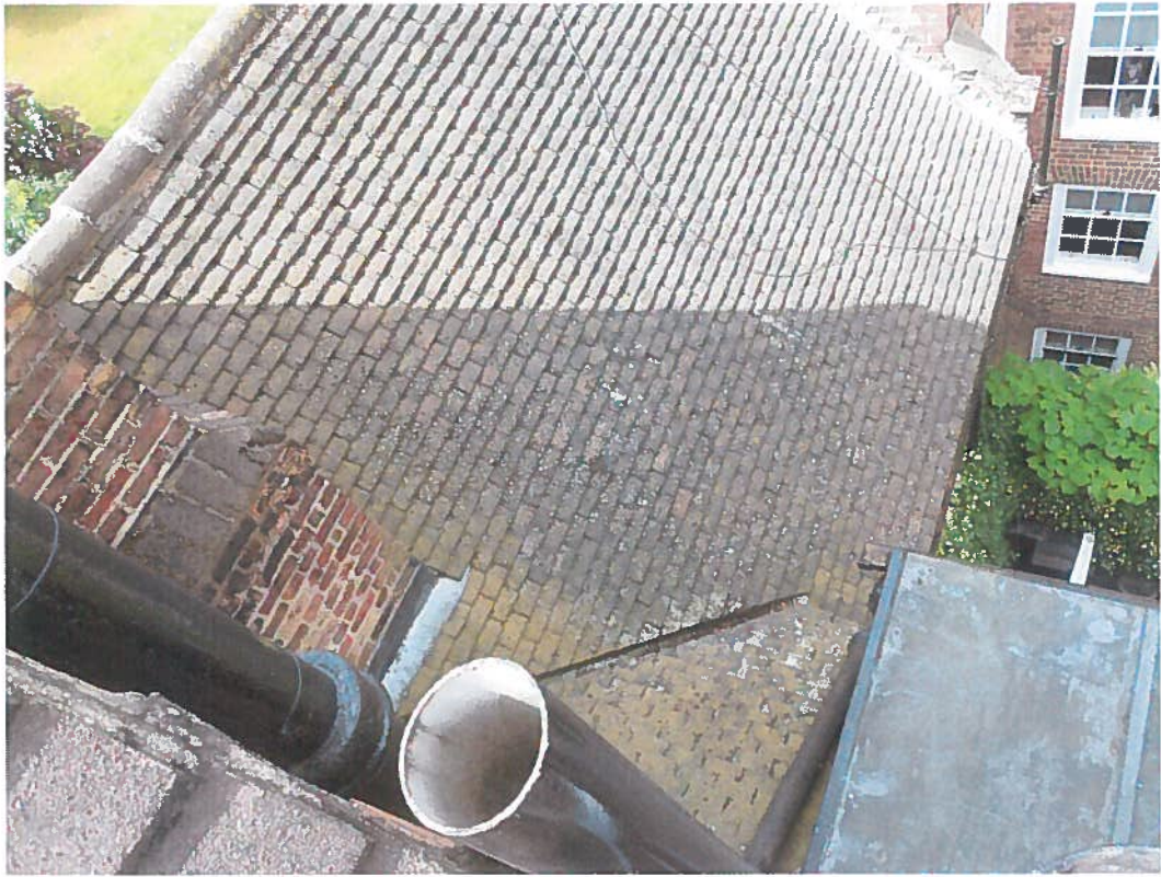
Photo 11 – Roof over annexe
