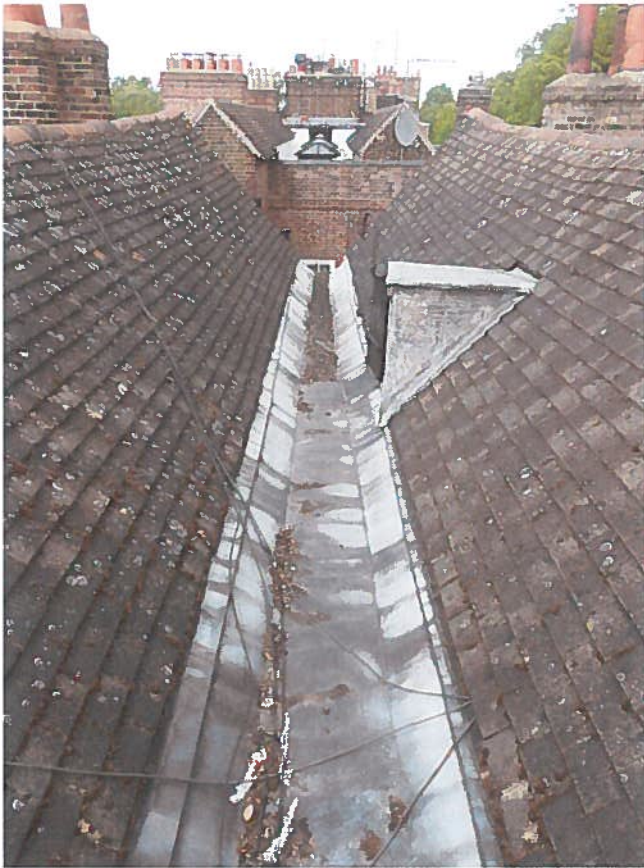
Photo 7 – Central valley to main roof
