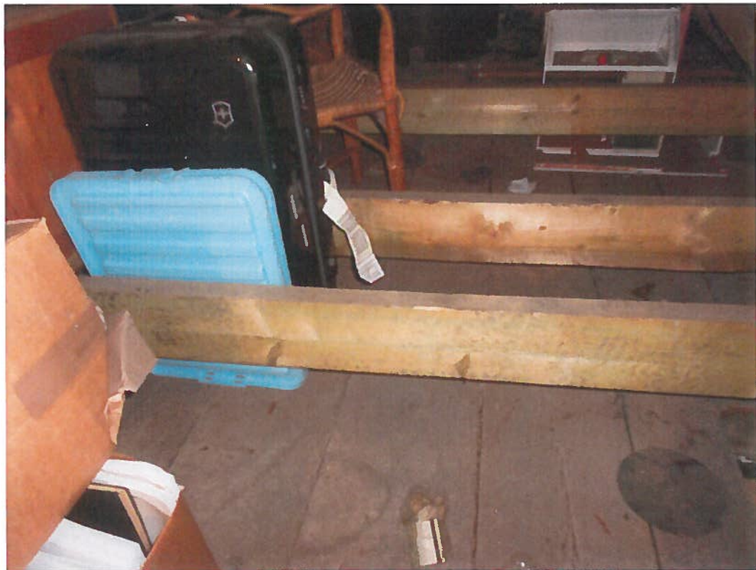
Photo 12 – New ties across rear pitch of main roof
