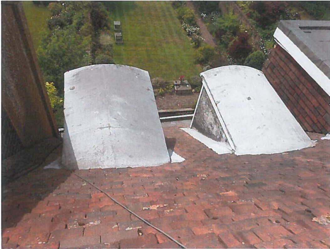
Photo 5 – Main roof – rear slope
