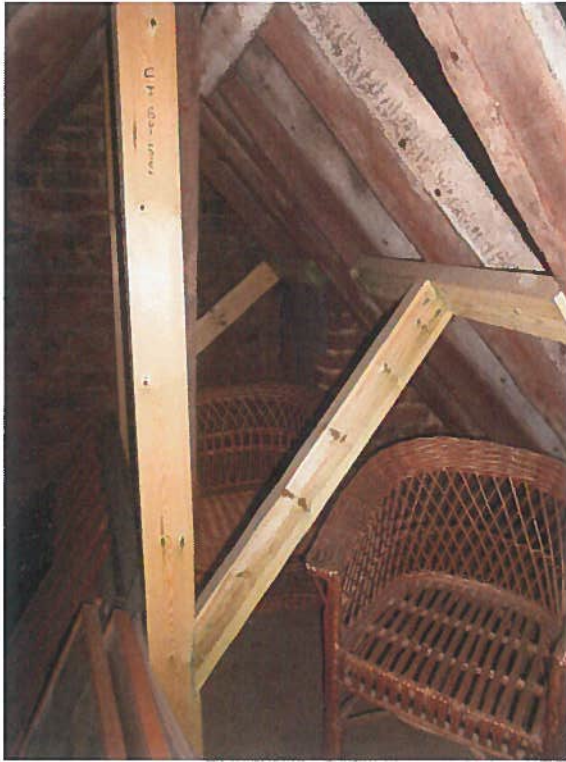
Photo 13 – New strutting to rafters of front roof pitch
