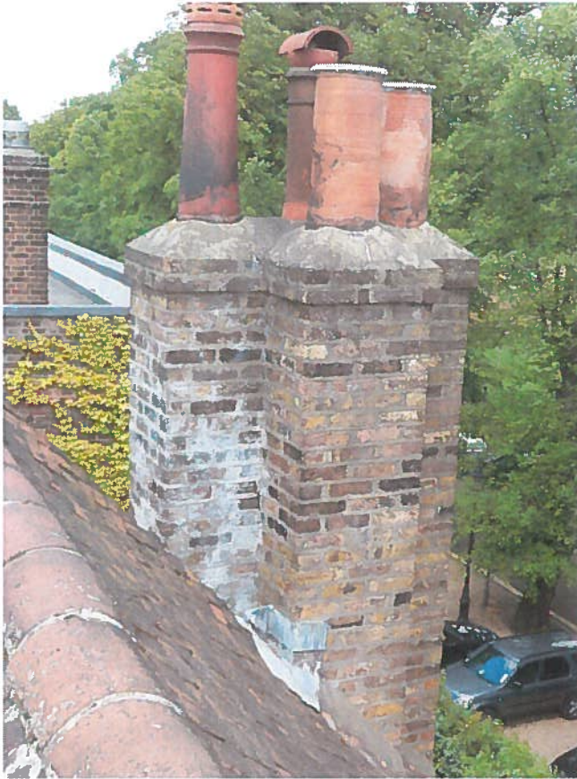
Photo 3 – North east chimney
