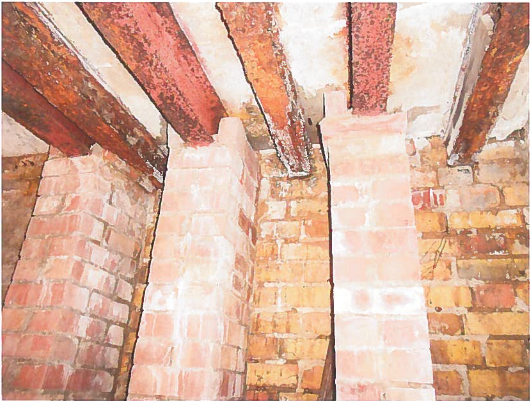
Photo 34 – Steel beams and brick piers in garden vault
