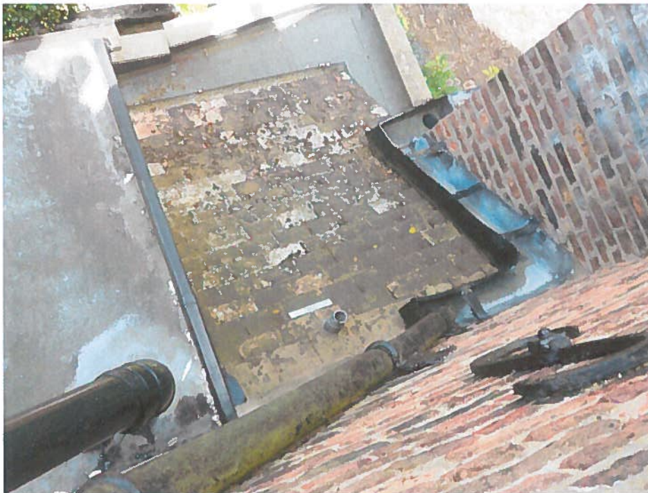
Photo 8 – Zinc flat and tiled lean-to roofs over north extension
