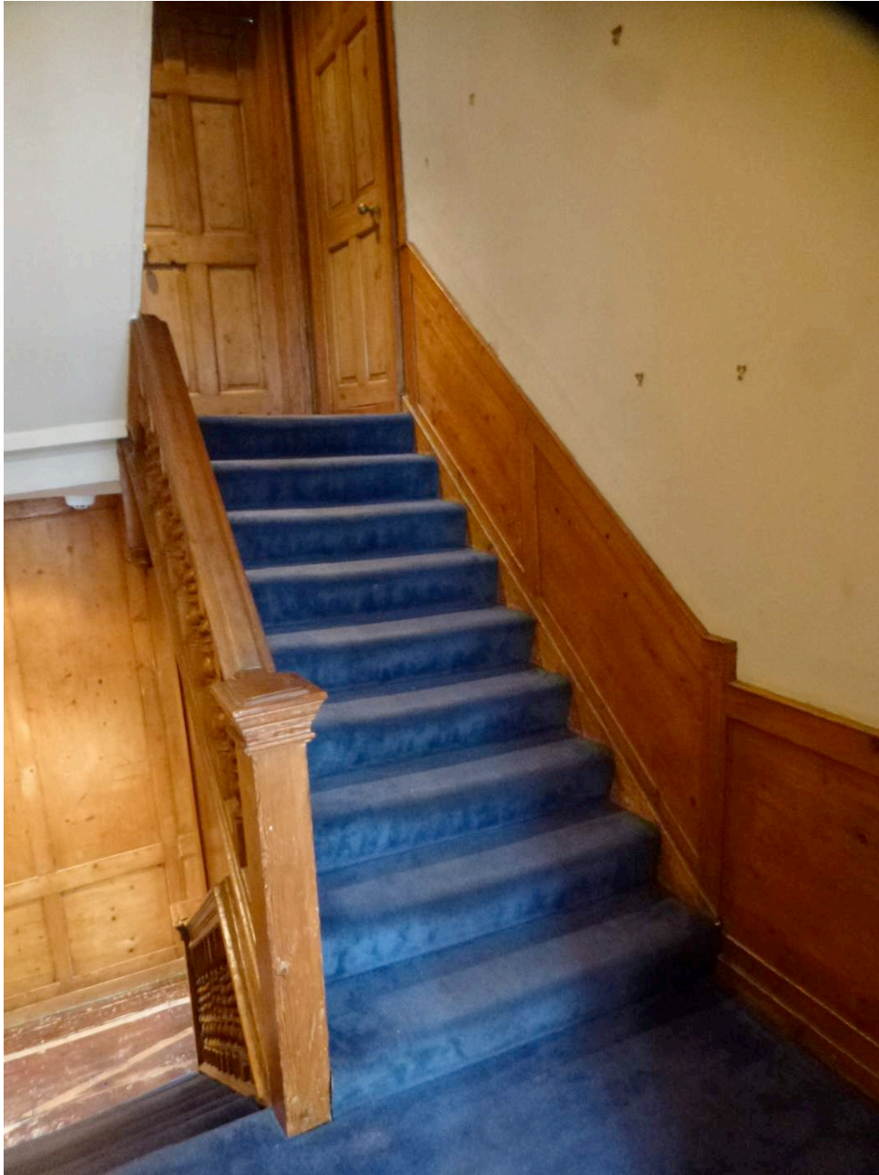
First Half Landing to First Floor Landing
