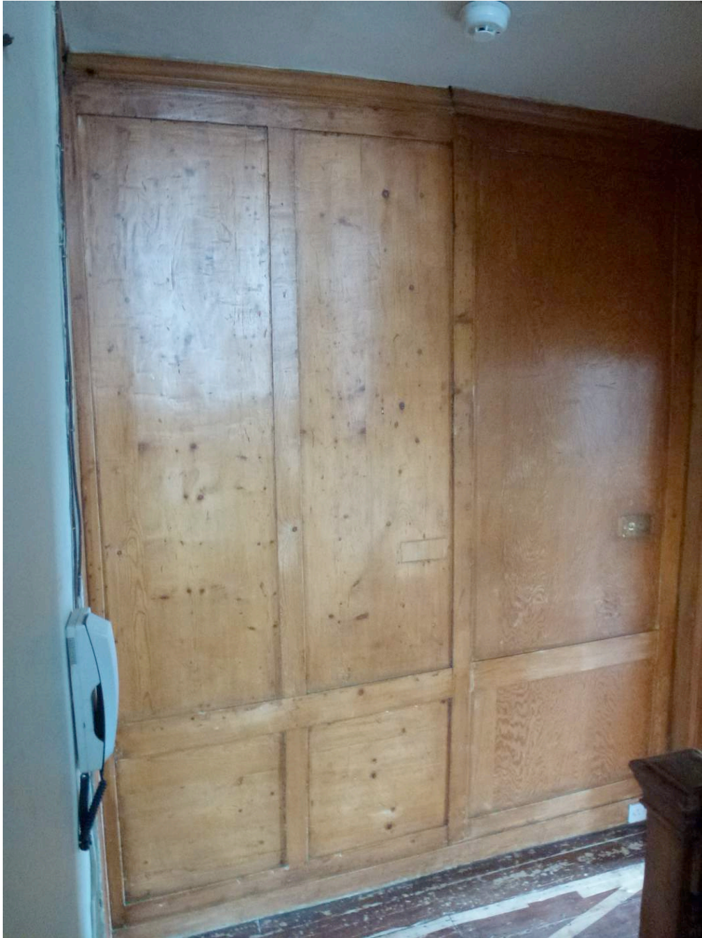
Panelling to Upper Ground Floor Landing
