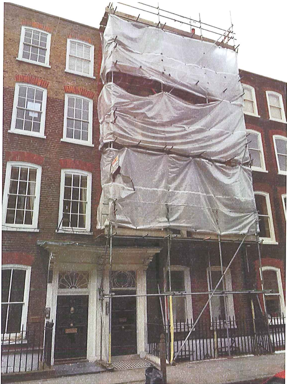
Photo F – Adjacent Building Which is Currently Undergoing Works
