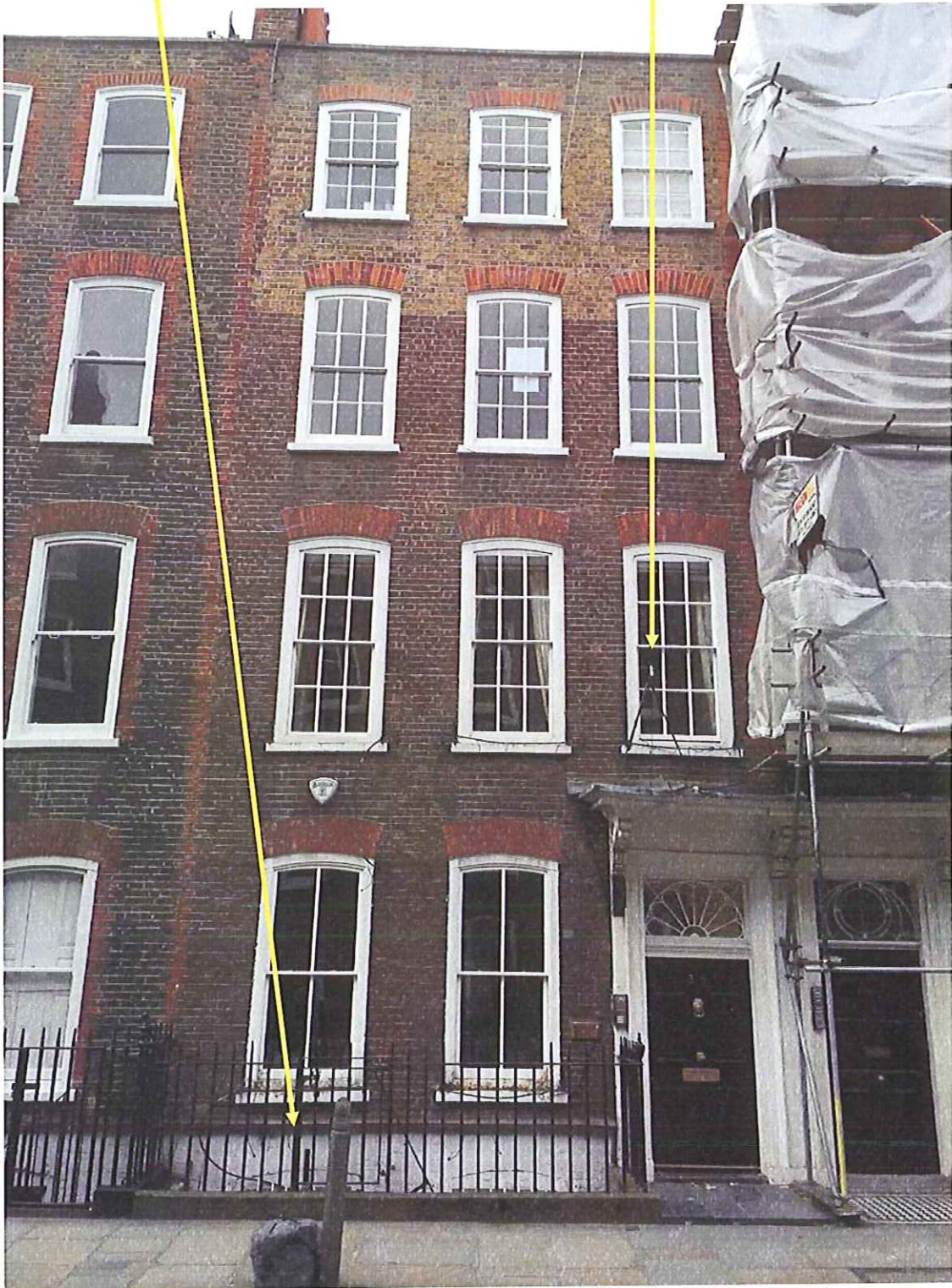
Photo A – Front of Building at 35 Great James Street with Microphone Located on Top of Entrance Canopy
