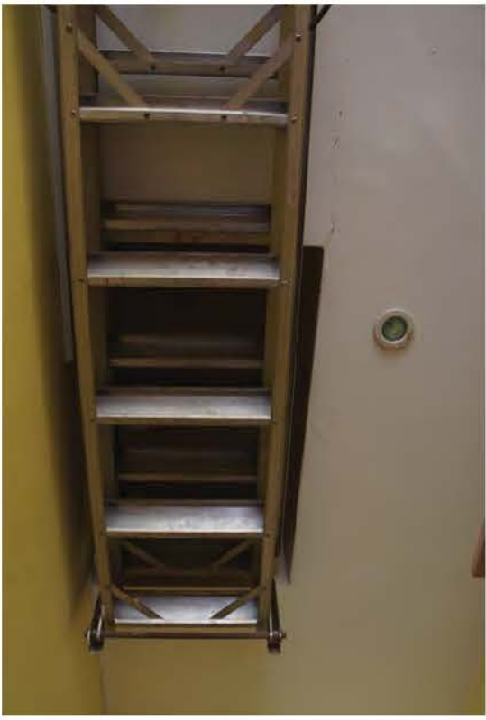
Ceiling - Roof Access Hatch
