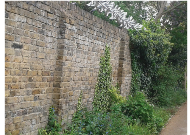
03 Existing brick wall to north side of private drive.
