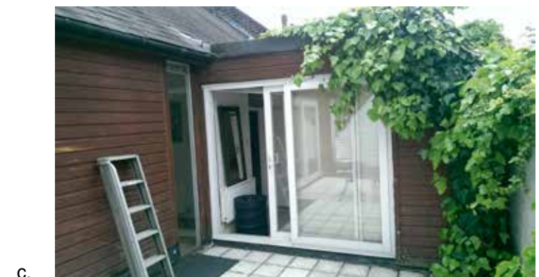
Figure 1a-c. Existing 1st floor roof terrace a. view looking towards No 10 b. view looking towards Daleham Gardens c. 1st floor bedroom addition from 1969 where the roof chamfers down to meet the top of the rear boundary wall.
