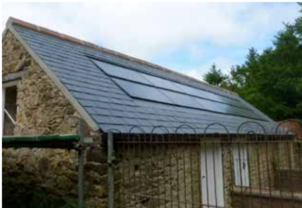
Figures 5a & b. Examples of in-line PV panels set flush into slates roofs.
