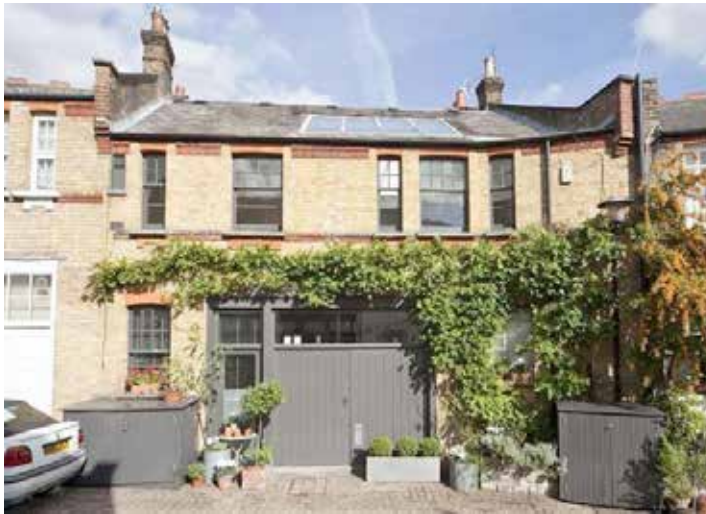
Figure 4. Large flush skylight currently at No 11 Daleham Mews.
